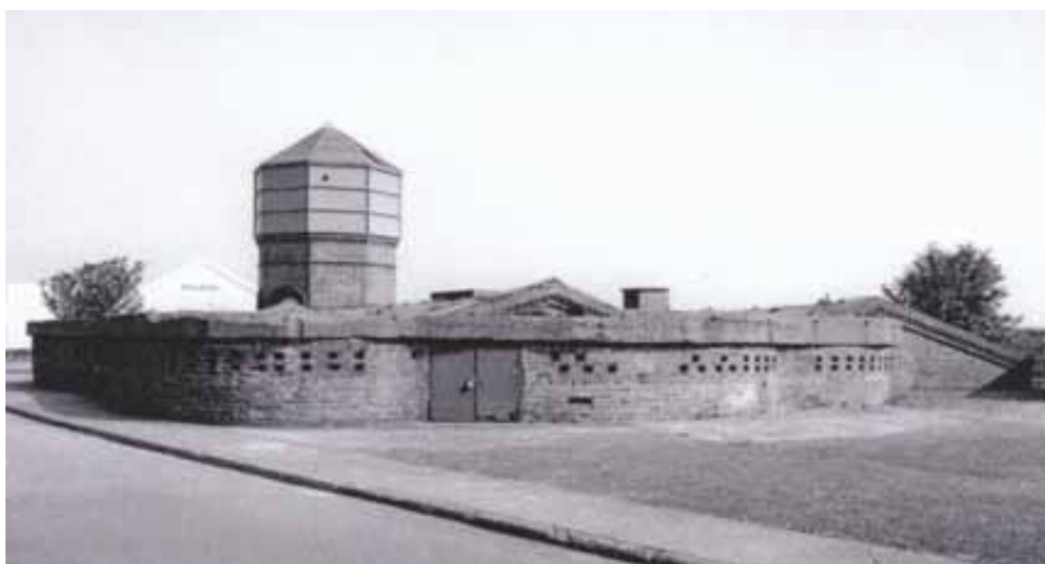
The Pump House, from the south, photo taken 1998 (NMR: AA043943); the high-level water tank shown was built in 1891
