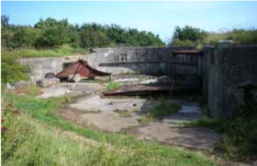
The Citadel Battery, emplacement III, photo taken 2011 (author)
