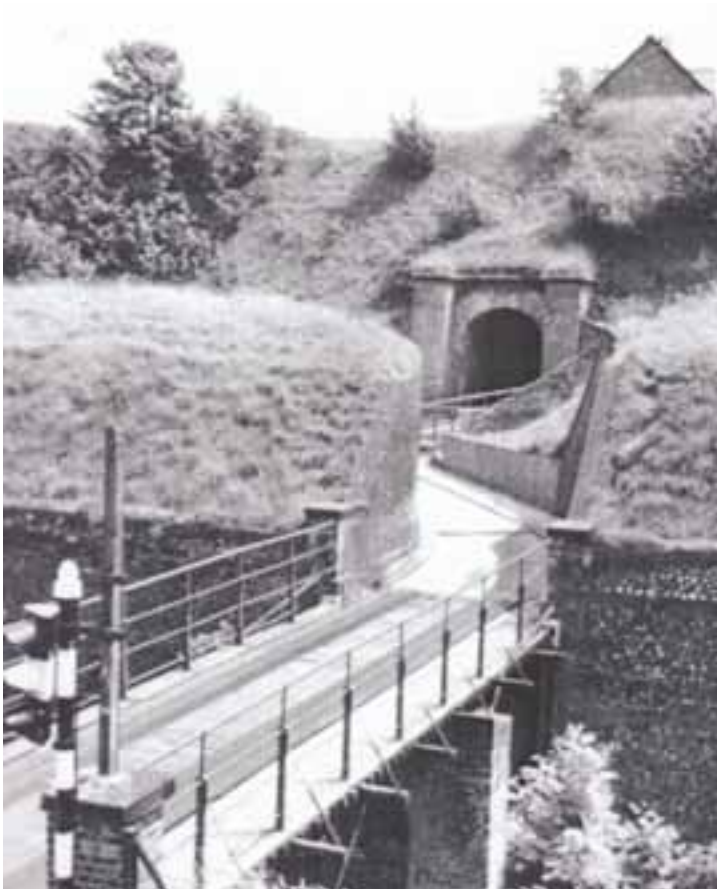
The North Entrance's outer entrance, photo taken 1958 (d07871 Dover Museum)
