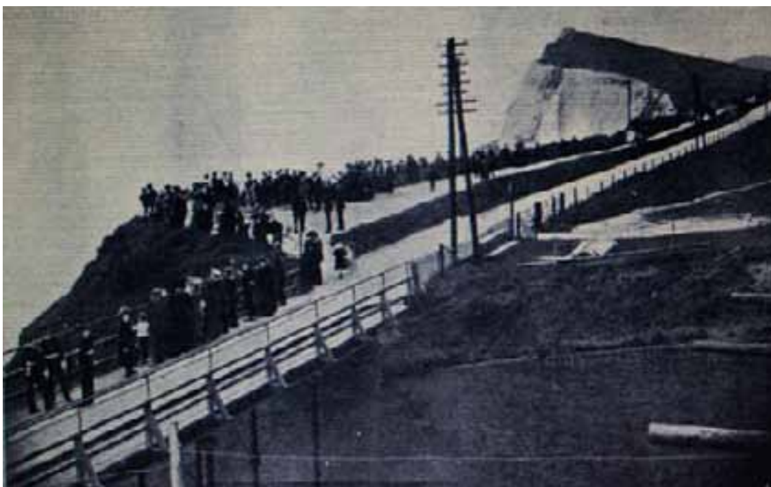
The South Lines Bridge, from the east, photo taken 25th July 1909
