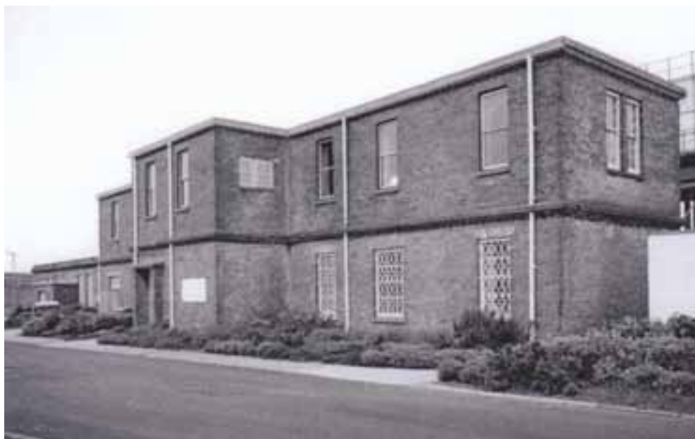
The Regimental Institute (former Canteen, then Recreational Establishment), photo taken 1998 (NMR: AA043938)
