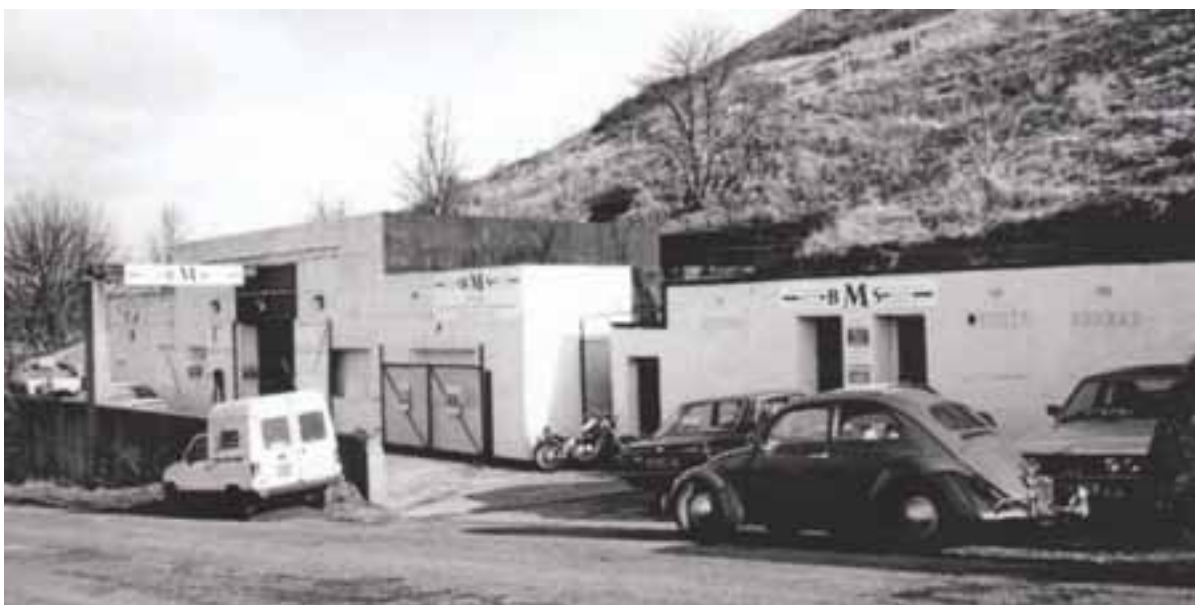
The REME workshop, from the north-west, photo taken 1998 (NMR; RCHME Report No. 10: Figure 20)
