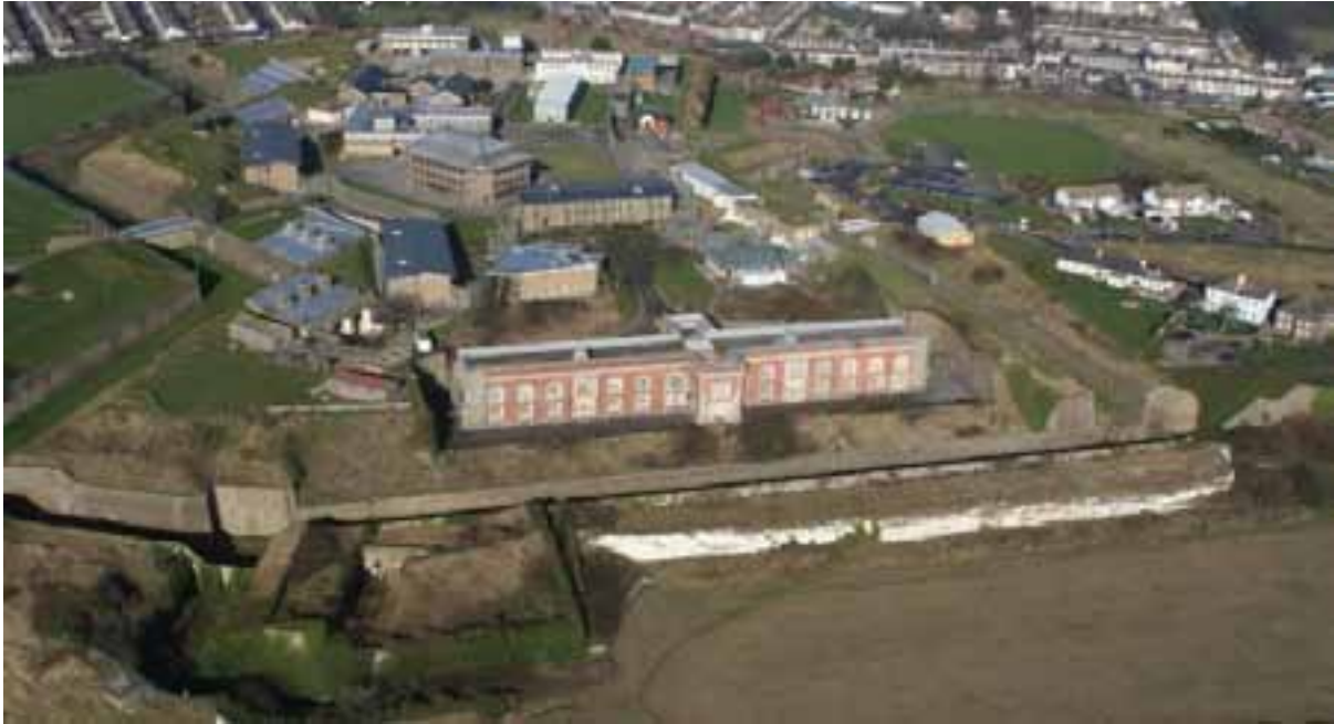
The Citadel, looking north, showing the Officers' Quarters (built 1858-67) in the foreground, and the post-1956 development on the Parade Ground, photo taken 2011 ( www.subterraneanhistory.co.uk )
