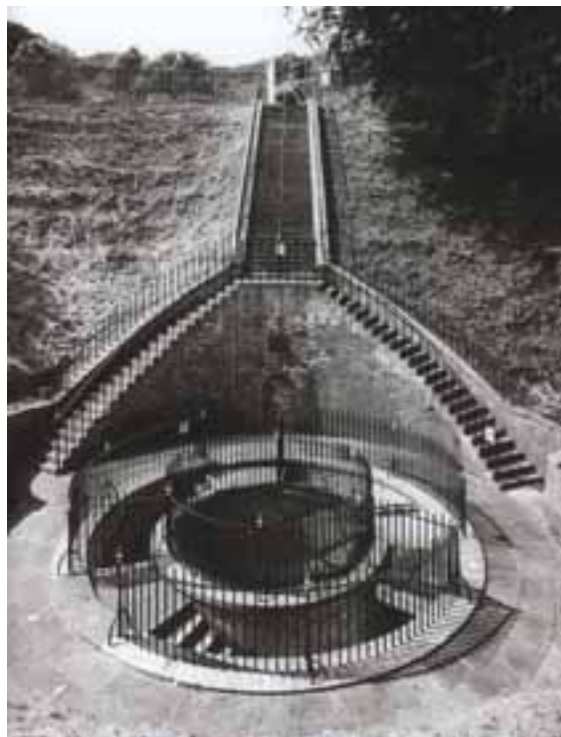
The steps from the Parade Ground down to the entrance to the Grand Shaft, photo taken 1998 (NMR: AA008568)
