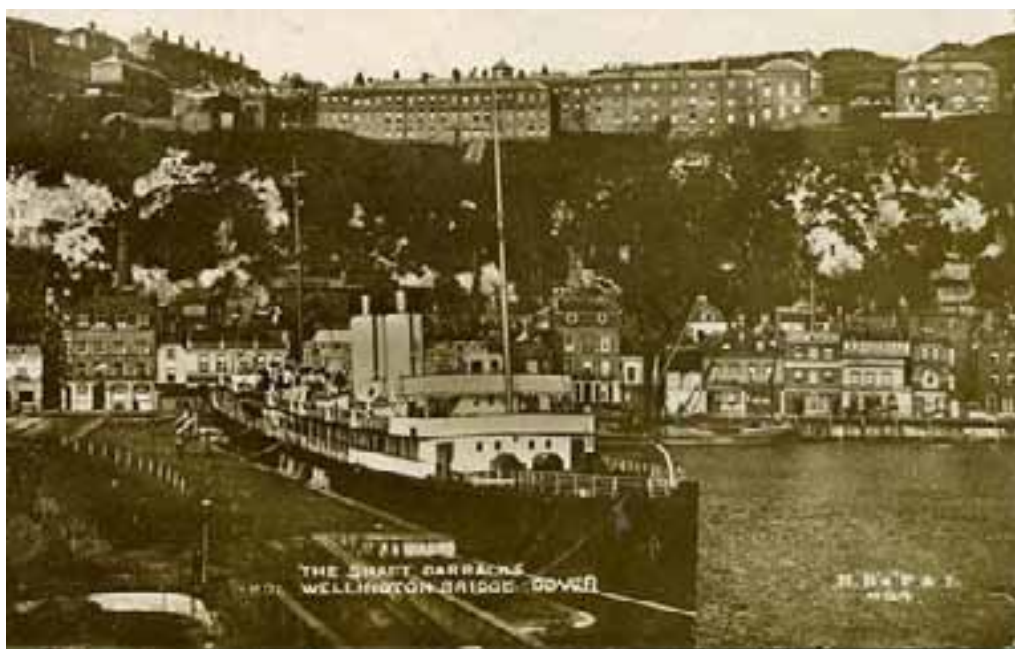
The Grand Shaft Barracks, from Wellington Bridge, postcard, late nineteenth/early twentieth century
