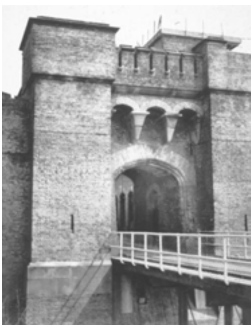
The South Entrance or Archcliffe Gate, photo taken 1958/9 (d07872 Dover Museum)
