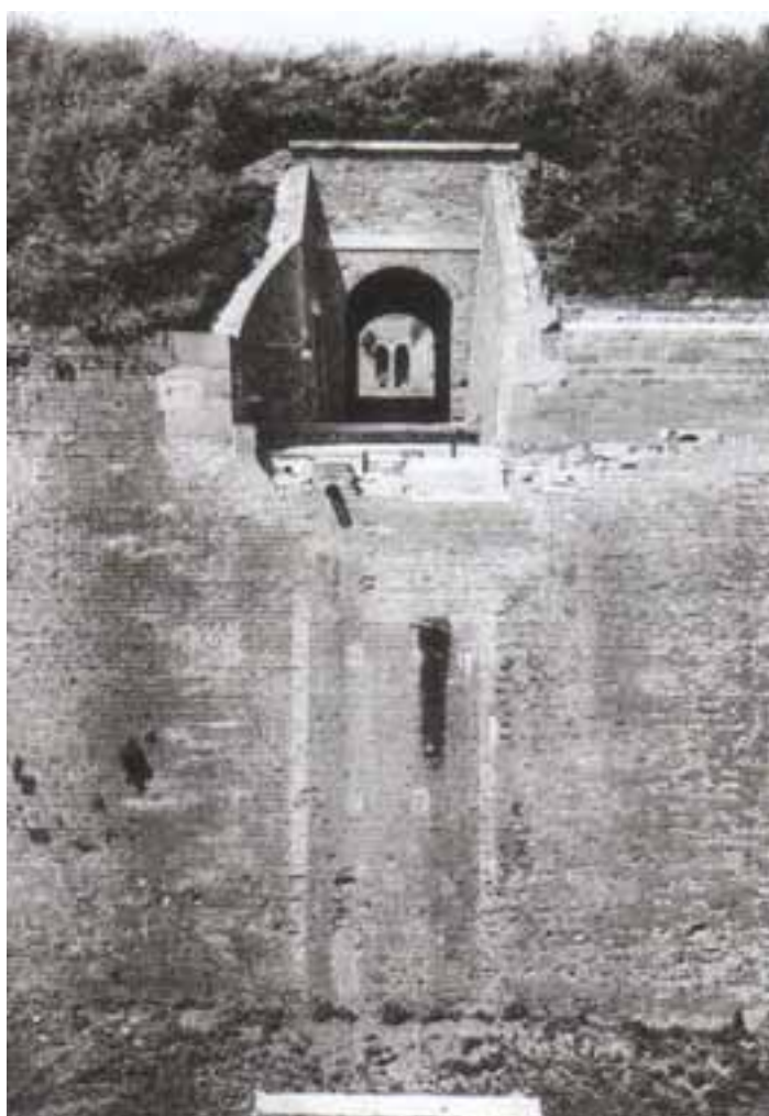
The Main Entrance in the southern face of the Drop Redoubt, looking north, photo taken 1998 (NMR: BB9915909)
