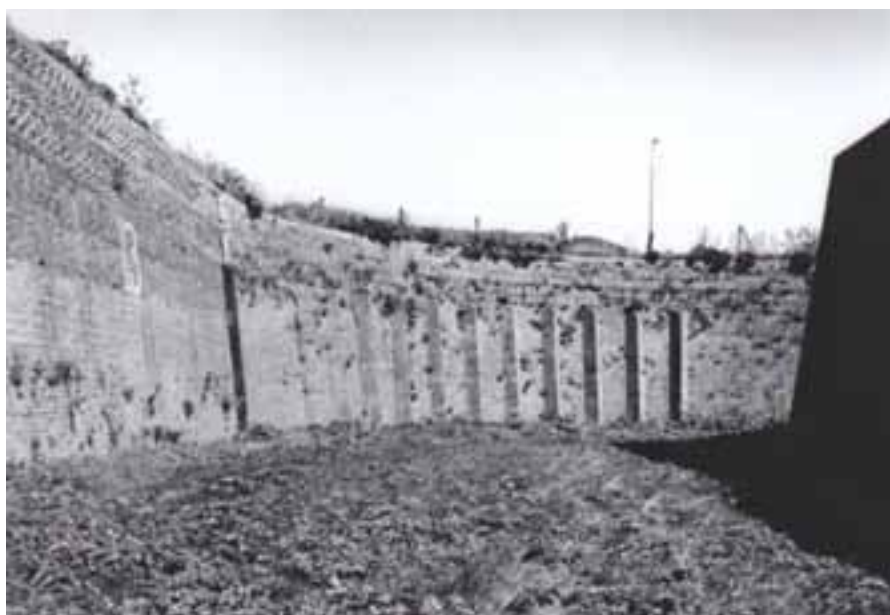
Anti-ricochet pilasters against the counterscarp of the Gorge Ditch, from the west, photo taken 1998 (NMR: BB032731)
