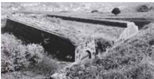
The Guard Room on the Centre North-West Bastion, from the south-west, photo taken 1998 (NMR: AA043948)
