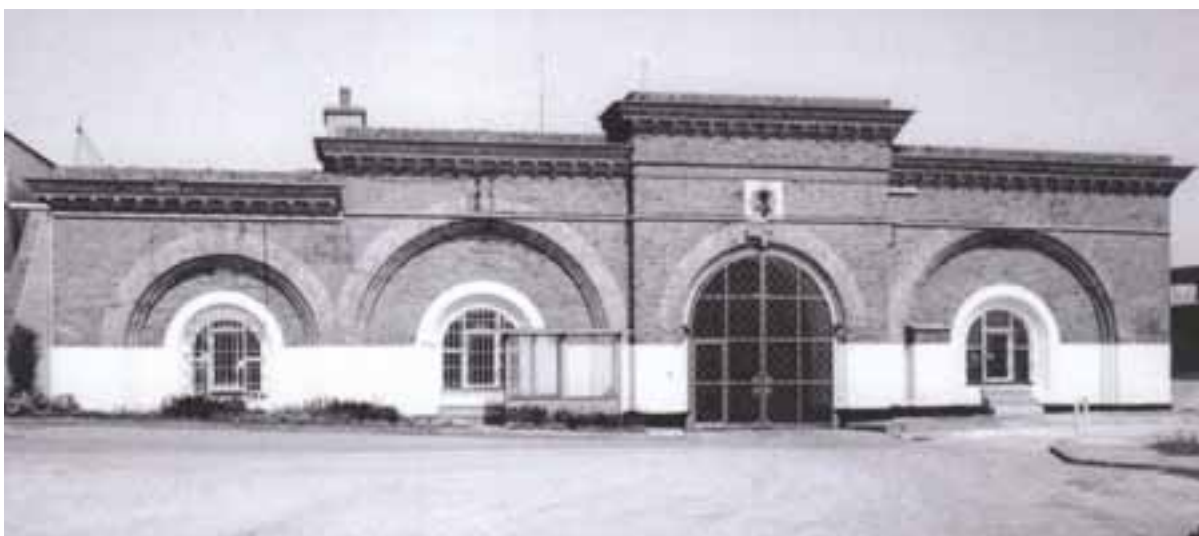
The Main Entrance in the Citadel, viewed from the Parade Ground, photo taken 1998 (NMR: AA043941)
