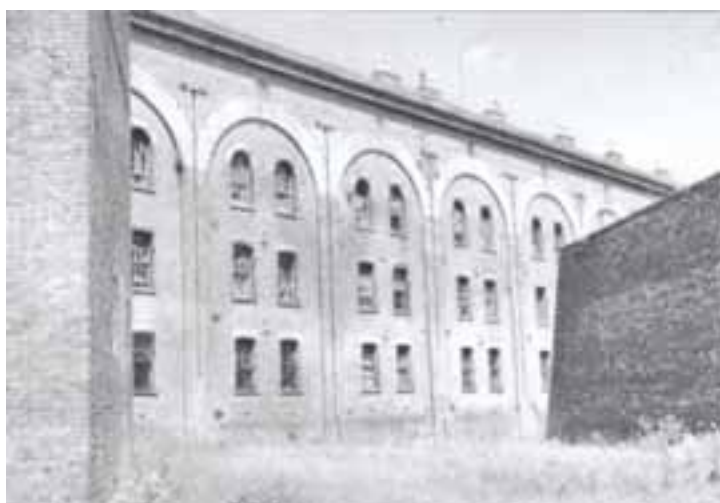
The casemated South Front Barracks, south-eastern elevation from the ditch, photo taken 1958/9 (d07879 Dover Museum)
