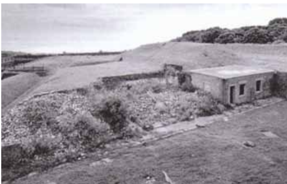
The twentieth-century shelter on the site of the western Staff Sergeants' Quarters, and the remains of the Ablution Room, Bath Room, Cook House, Latrines and eastern Staff Sergeants' Quarters demolished after the Second World War, photo taken 1998 (NMR: BB99/15932)
