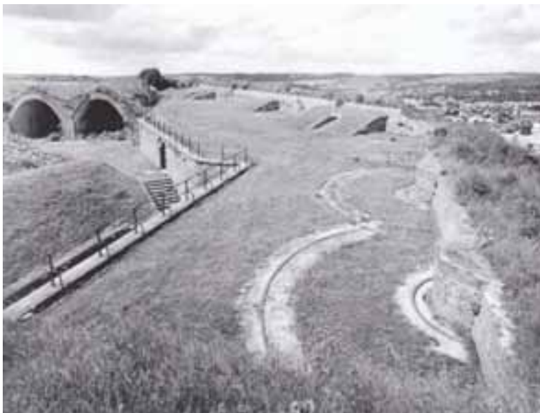
The Drop Redoubt's terre-plein along the eastern and the north-eastern faces, showing the parapet, gun emplacements and racers for traversing platforms, photo taken 1998 (NMR: BB99/15925)
