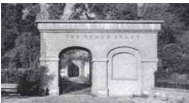
The recreated lower entrance (gateway and Guard Room) to the Grand Shaft, photo taken 1998 (NMR: BB013811)
