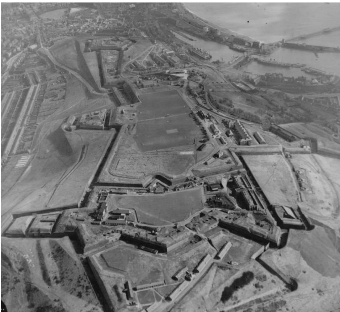
The Western Heights, from the west, photo taken 1939; the remains of the South Front Battery (south of the Citadel's tenaille) are visible on the right
