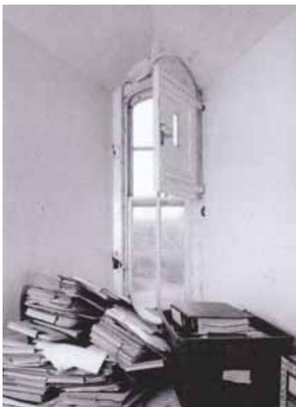
Officers' Quarters, armoured shutter to a first-floor window on the northern porch's western elevation, photo taken 1998 (NMR: AA043959)
