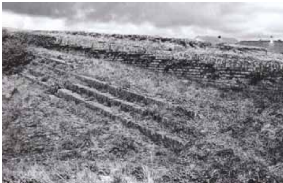
Banquette at the southern end of the gorge rampart, from where the approaches to the Citadel's Main Entrance were defended, photo taken 1998 (NMR: BB032736)
