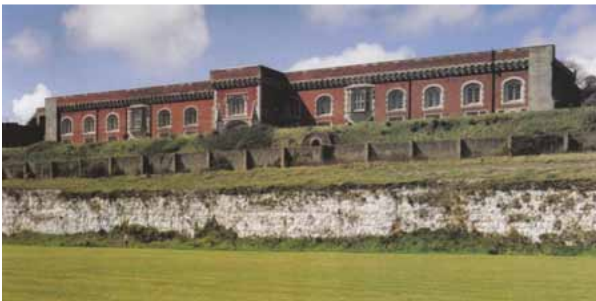
The southern (original front) elevation of the Officers' Quarters in the Citadel, photo taken 1998 (NMR: BB032722)
