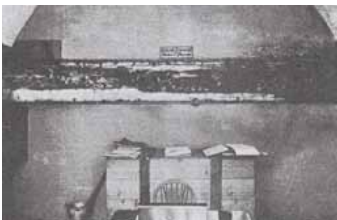
The foundations of the pharos visible in the rear wall of casemate 6 of the Officers' Quarters at the Drop Redoubt, photo taken c. 1891 (Wheeler 1929: Plate XIII A)
