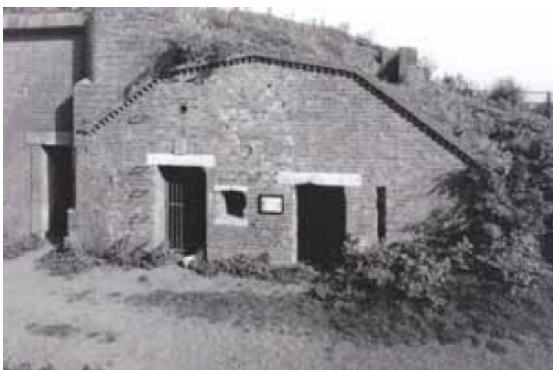
St Martin's Battery, showing the doors to the lamp store (right) and shell store A, with the lamp recess between them, photo taken 1998 (NMR: AA9909711)
