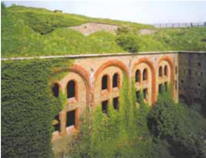
The South Flank Casemates, from the south, photo taken 1998 (NMR: BB032747)
