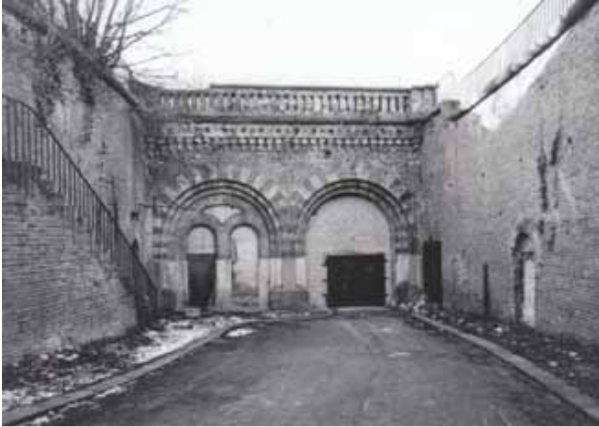
The front elevation of the North Entrance's inner entrance, looking northwards along the deep cutting, photo taken 1998 (NMR: AA00/9818)
