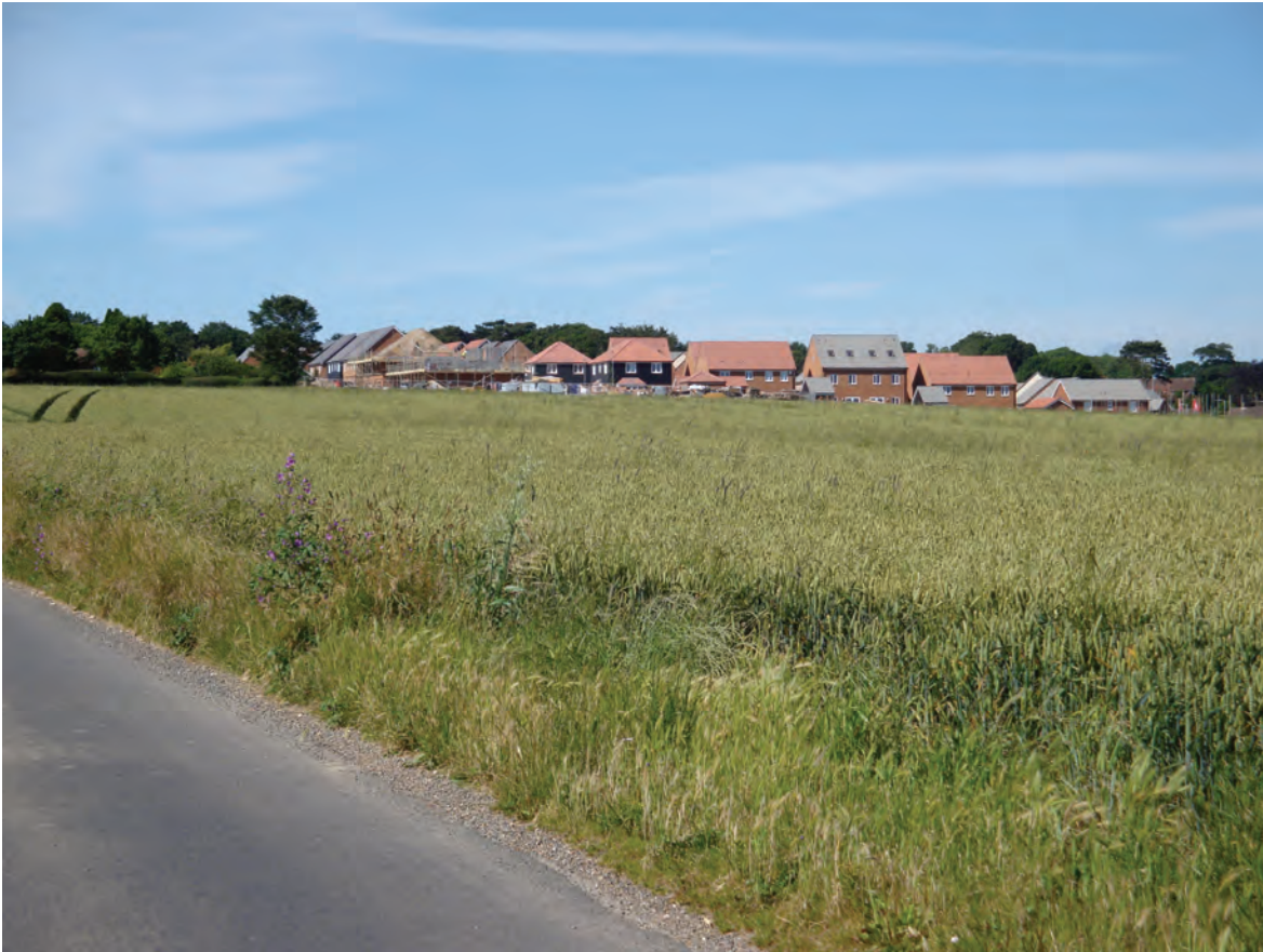
Figure 11.3 Image of Abbey Homes development, Whitfield taken from Napchester Lane
