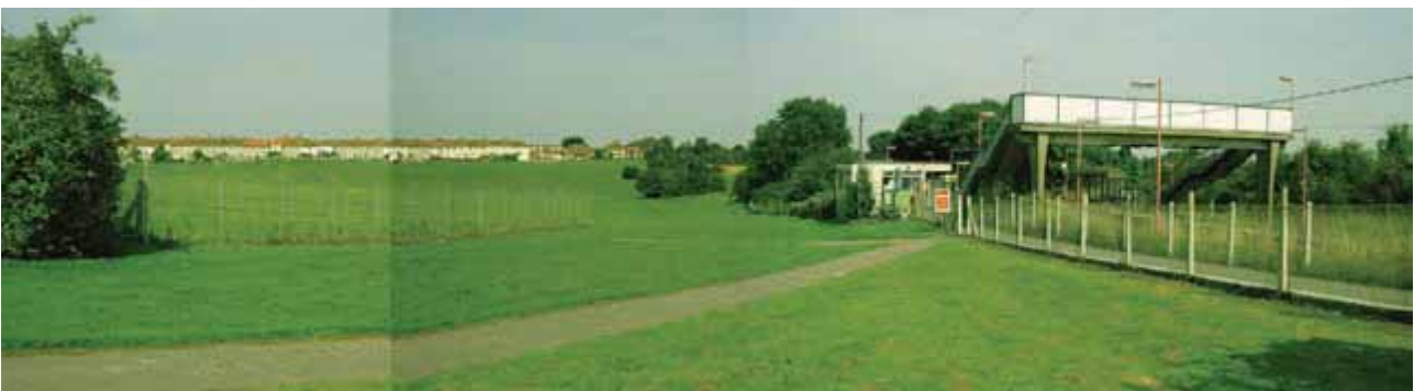
Poor pedestrian access to Aylesham station
