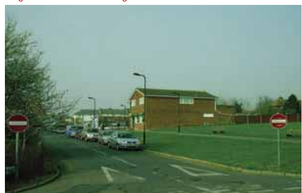
Existing post office buildings
