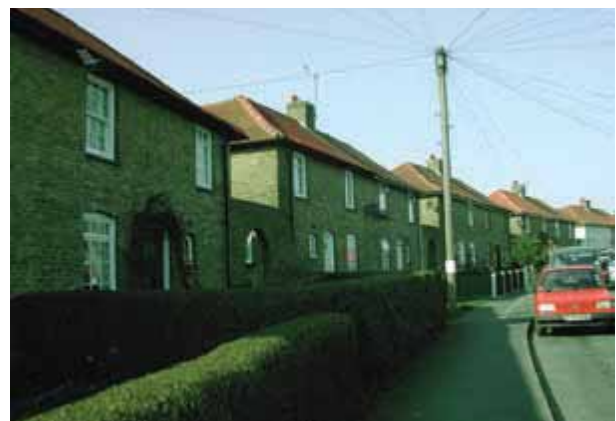
Original Abercrombie buildings
