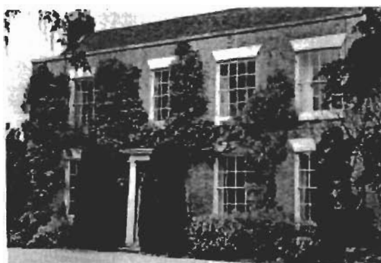
Forstal House: Late Georgian stock brick façade with parapet fronting earlier 17 th C farm cottage
