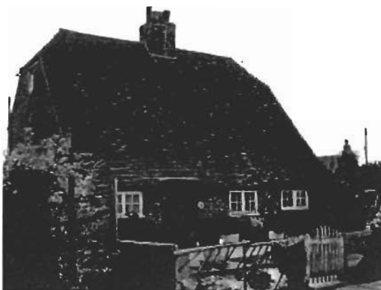
Padbrook Cottage: early 18 th C cottage with long "cat's slide" roof
