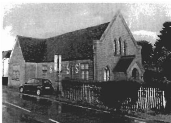
The former Chapel, 1825 & 1836, now a private house
