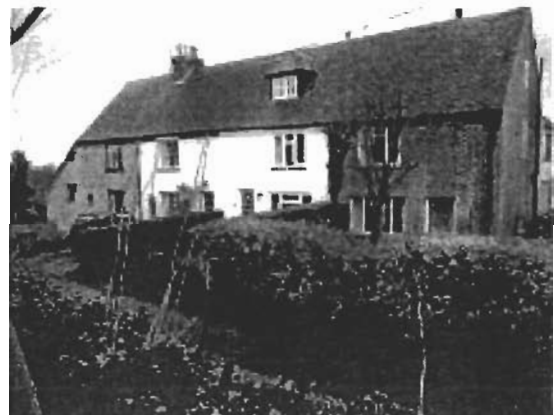
Speedwell Cottages, the former Workhouse
