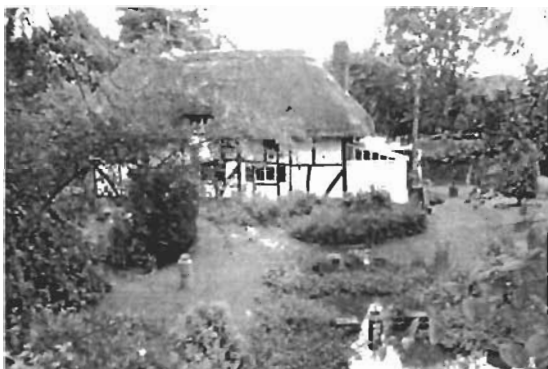
Ivy cottage 16 th C Timber frame cottage with long straw thatched roof
