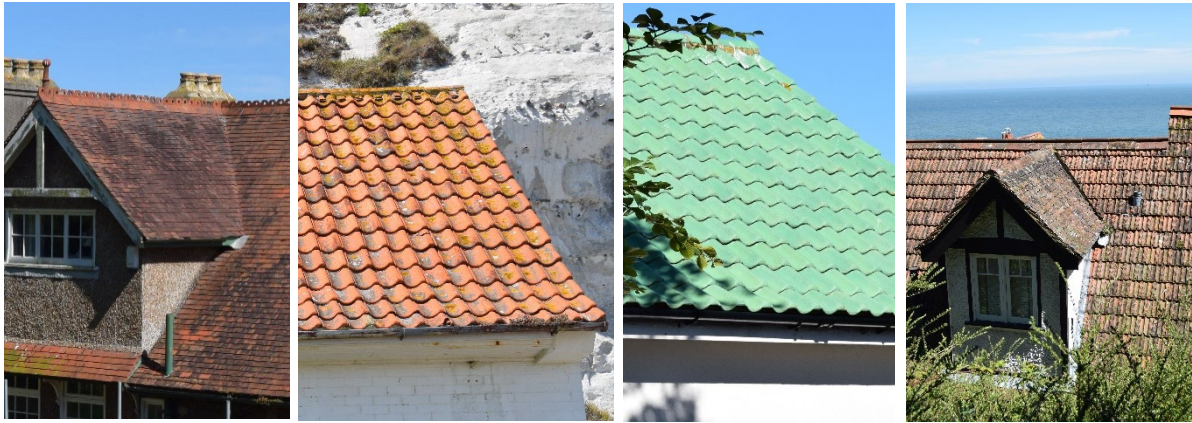
Left to right: plain tiles, pantiles, glazed pantiles and interlocking clay tiles
