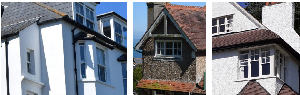
Examples of smooth render (left), roughcast render (middle) and painted roughcast (right)
