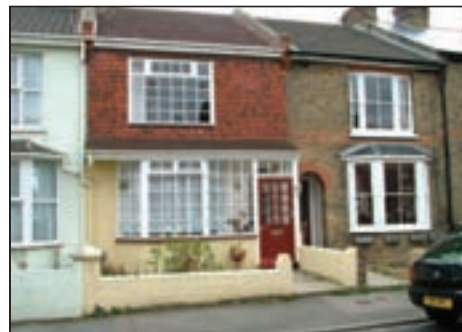
Enclosed arched doorways, Downs Road
