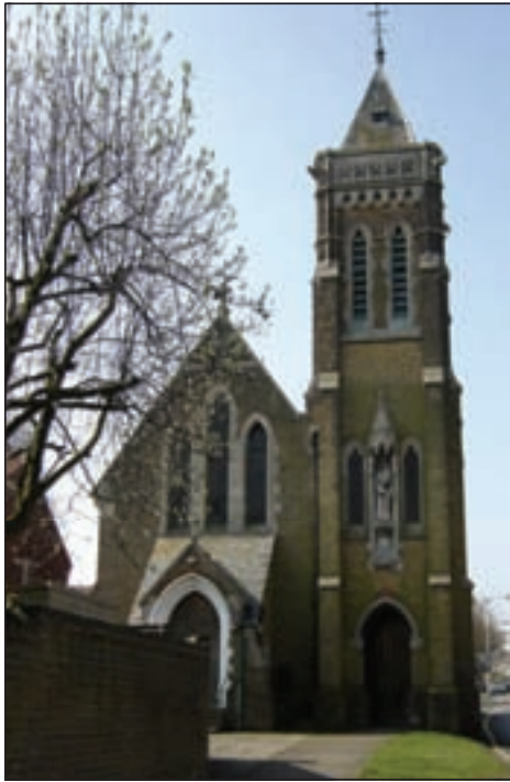
Pugin designed chapel, Dover Road (listed)
