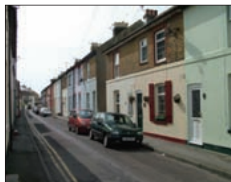
Small terraces, Campbell Road
