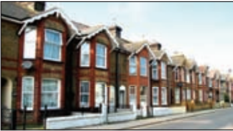
Brick terrace, Blenheim Road
