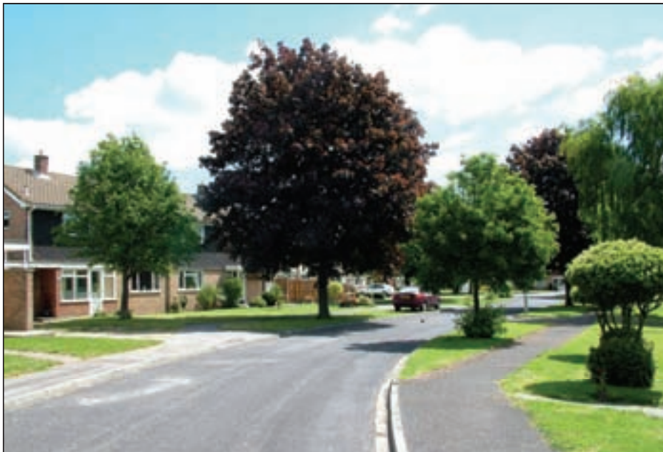
Former military housing, York and Albany Close
