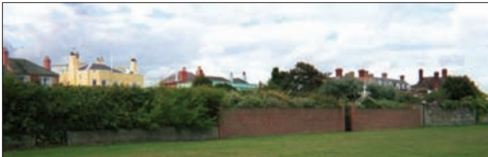
Private walled gardens on Walmer Green belonging to substantial properties on The Beach
