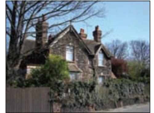
Rubble brick house, Dover Road
