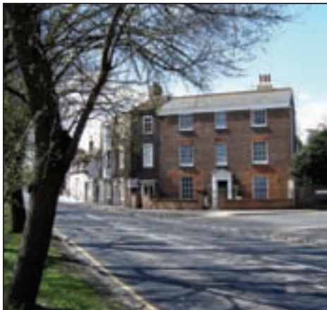
Large house, Church Street & Dover Road
