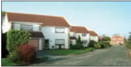
Positioned for solar panels, Whiteacre Dr.
