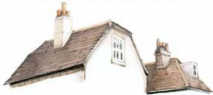
Georgian hip and half-hipped roofs, Dover Road
