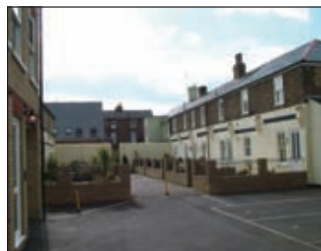
Infill terraces off Cambridge Road
