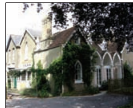
Gothic House, Dover Road (listed)
