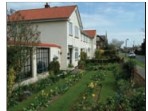
Linking walls, Palmerston Avenue
