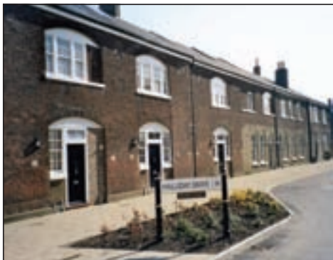
Original stables, Cavalry Barracks (listed)
