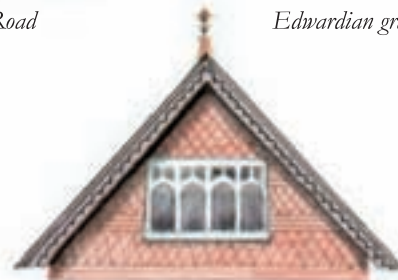
Edwardian tile hung gable, Dover Road
