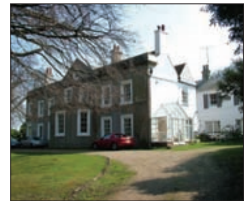
Liverpool House, Liverpool Road (listed)
