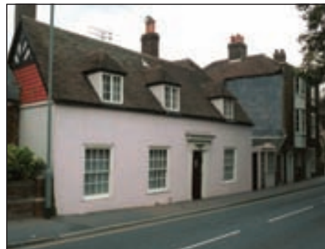
West side Dover Road near Church Street
