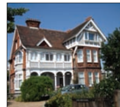
Porches and balconies, Marine Road
