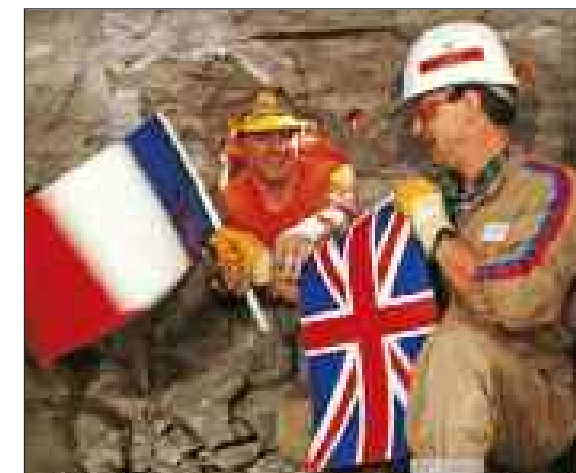
French and British Channel Tunnel excavations meet
