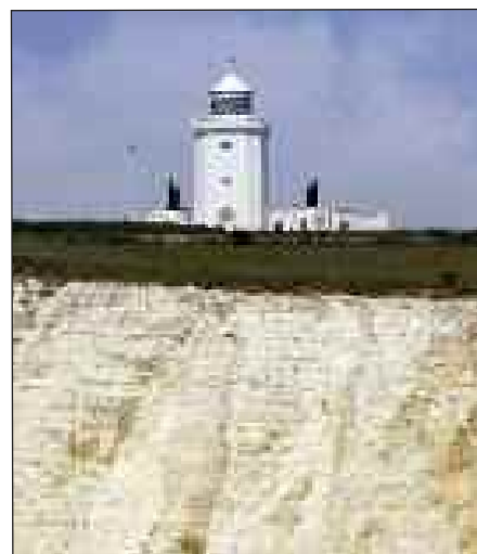
South Foreland Lighthouse
