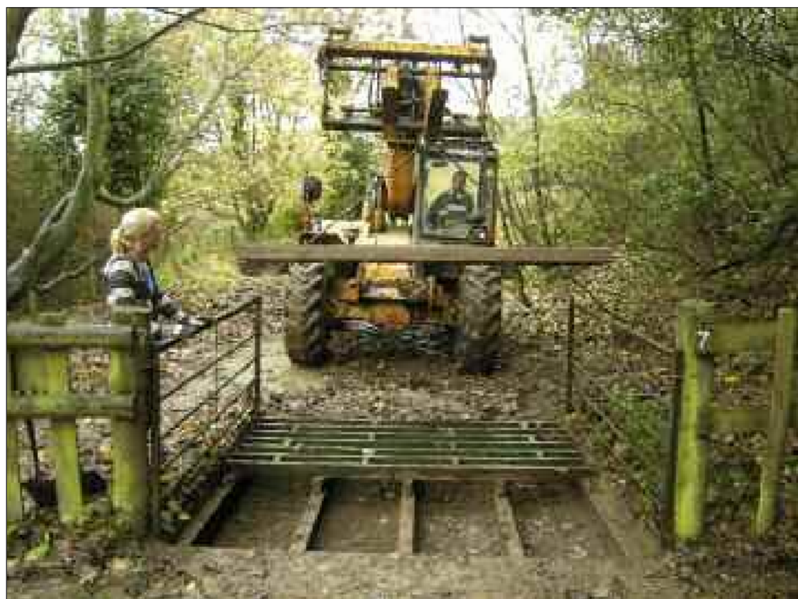
Lifting and cleaning a cattle grid
