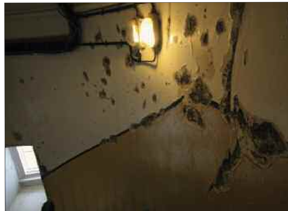
The deteriorating condition of the lighthouse
