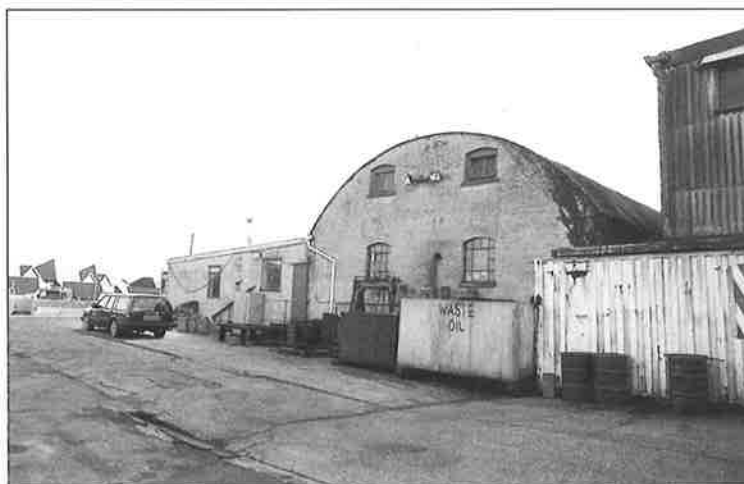
Interior of the Puma Manufacturing site
