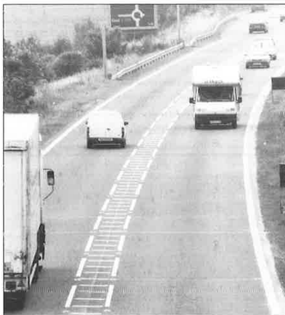
Single carriageway section of the A2
