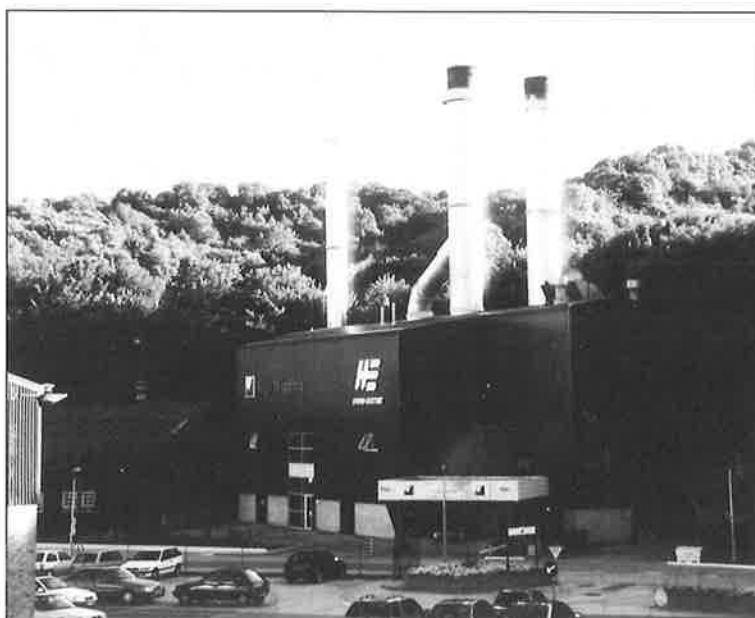
Combined heat and power plant, Dover
