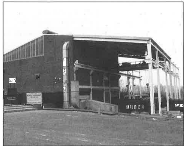
Waste Transfer Station, Whitfield
