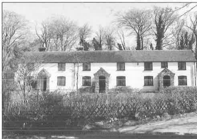
Domestic extension giving appearance of a 3rd cottage
