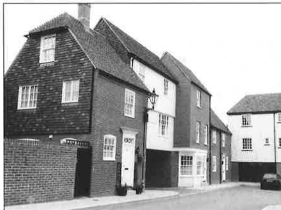
Development in Sandwich Walled Town Conservation Area
