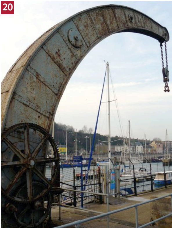
20. The Fairburn Crane, Dover Harbour
