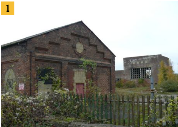
1. Disused buildings at Snowdown colliery.
