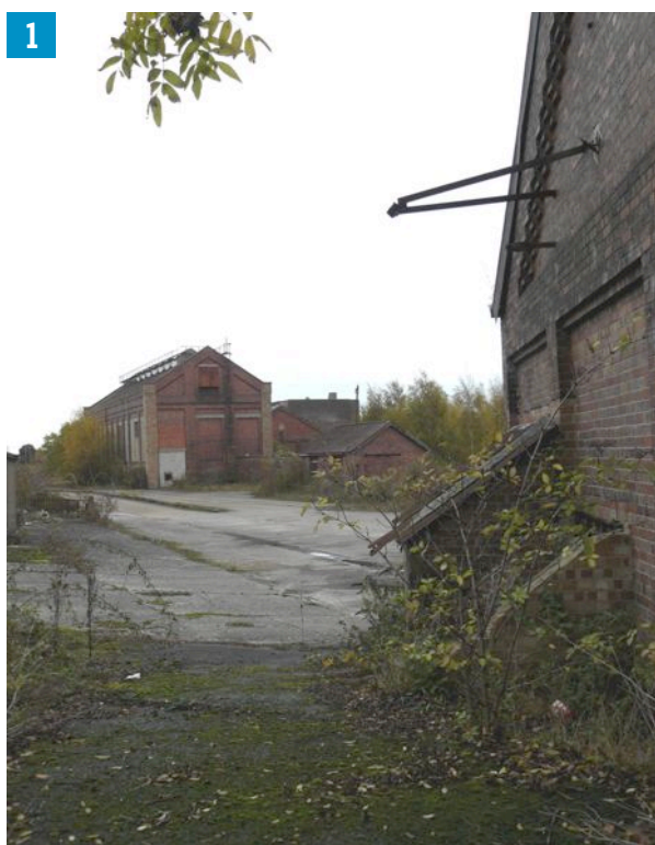
1. Derelict colliery buildings at Snowdown.
