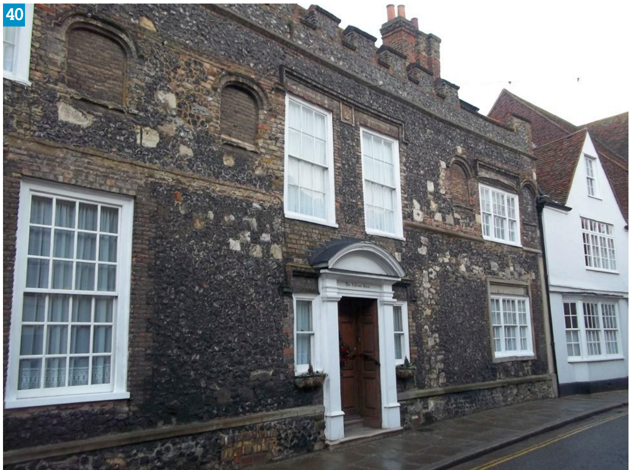
Figure 40 Pelican House, Sandwich exhibits a fine flint facade
