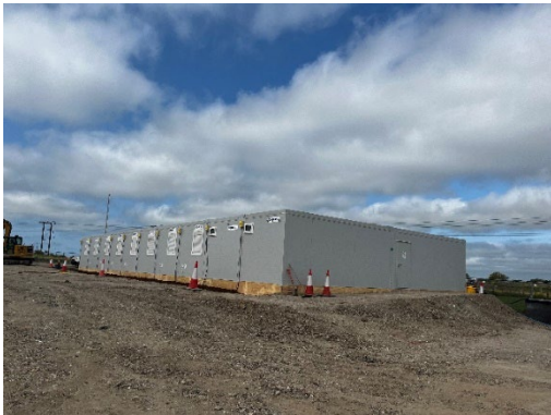
Image: New cabins for the temporary Colas site compound in Section 2.
