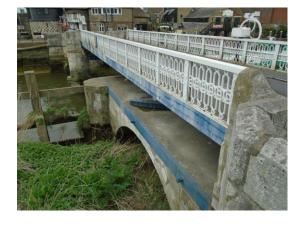
The bridge deck will be removed and transported to a yard to facilitate the works. The mechanical and electrical components at the bridge site and on the deck will be replaced and the opportunity will be taken to clean and repaint the bridge deck for maintenance purposes.
