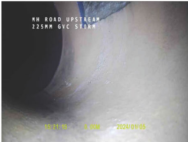
5, 00:00:09, 10.70 m Finish node type, manhole, reference number: MH1
