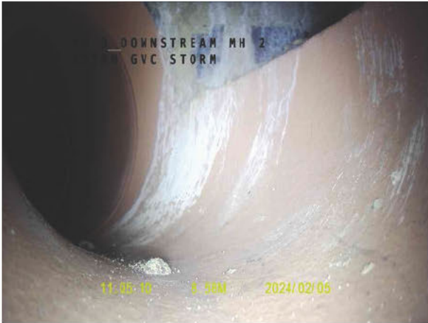
1, 00:04:29, 8.50 m Finish node type, manhole, reference number: MH2
