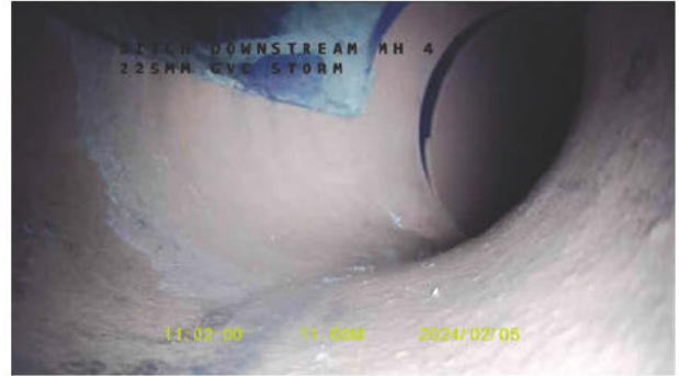
6, 00:02:48, 11.50 m Finish node type, manhole, reference number: MH4
