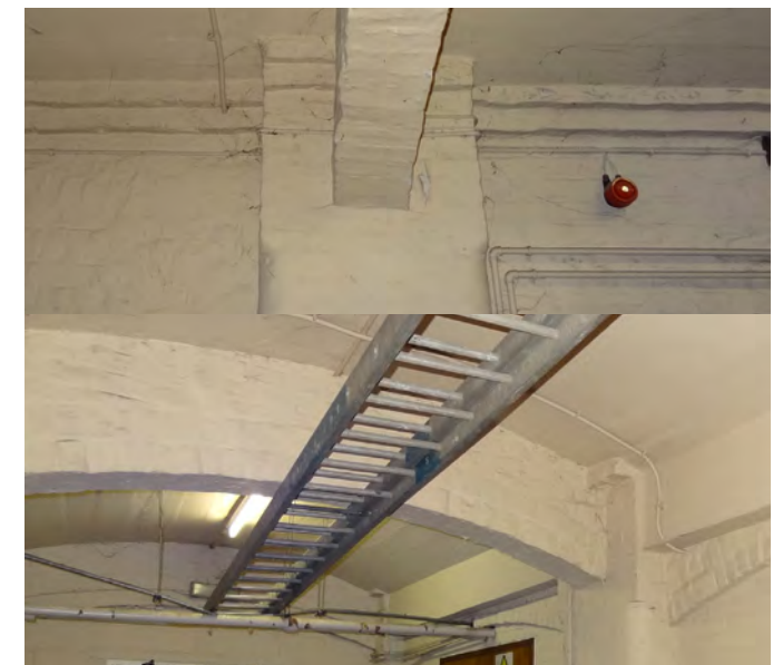
(h) Arched vaults & brick piers beneath Connaught Hall (Internal ref: DSC05485 & DSC05484)
