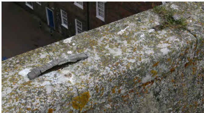
(i) Iron cramps to top of Tower parapet denoting Victorian repairs (Internal ref: IMG_4916)
