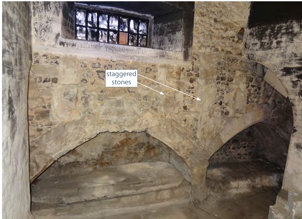
(c) Vertically stacked, staggered stones on wall face may indicate engaged columns for arcade or tomb canopy. (internal ref: DSC05498)
