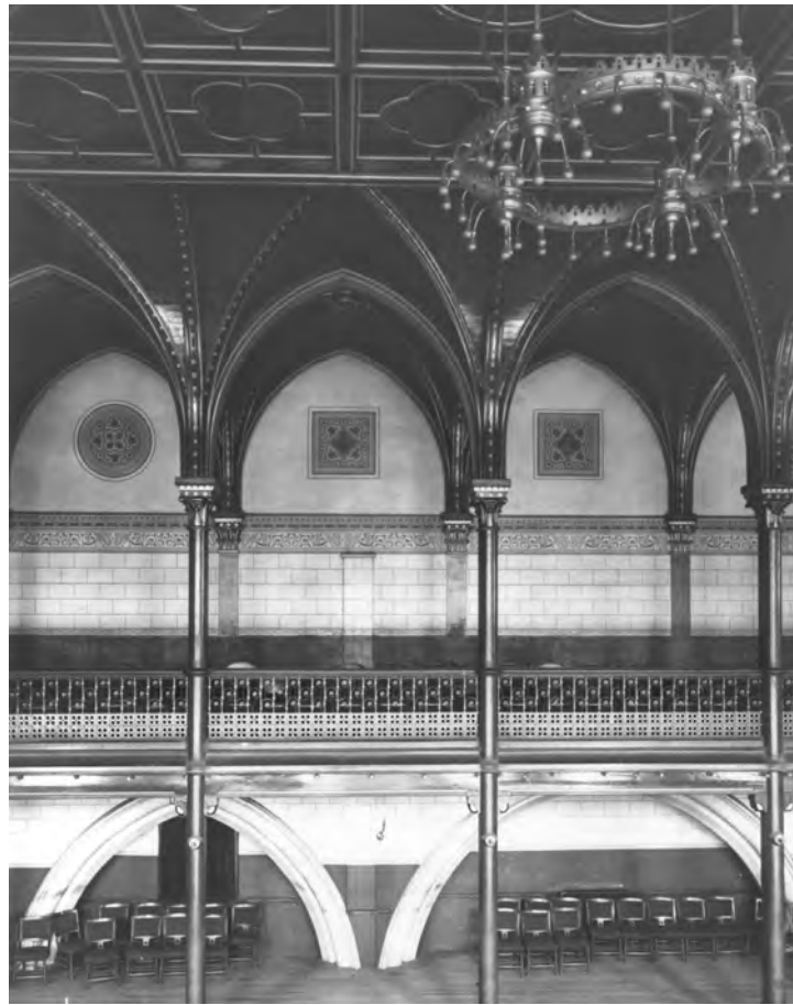
(a) South wall of Connaught Hall showing medieval arches and original decoration. (DMA ref: D44455)
