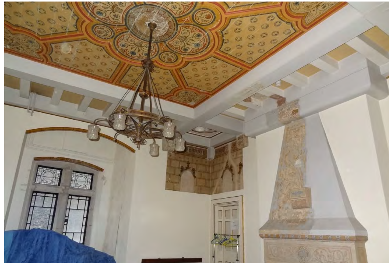
(c) Ceiling, chandelier, fireplace, infilled niches and uncovered decorations to Mayor's Parlour (Internal ref: DSC05067)
