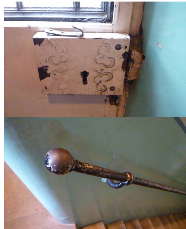
(e) Detail of original fixtures and fittings (Internal ref: P1120637 & P1120636)
