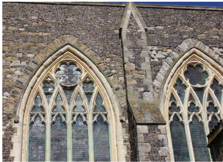
(b) The alternate Poynter tracery within early window surrounds. (Internal ref: IMG_5907)
