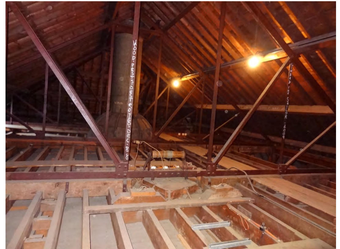
(c) Roof space above Connaught Hall. Note industrial iron girder structure and Sun Burner funnel in the background. (Internal ref: DSC04999)
