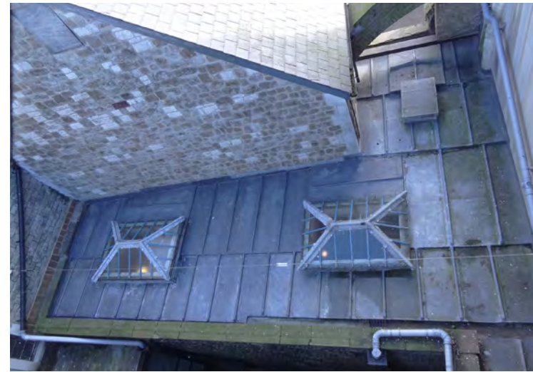
(b) Lead roof to anti rooms (Internal ref: DSC05585)
