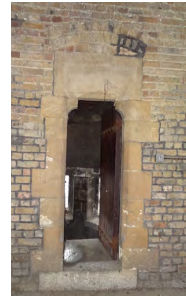
(f) Door to Tower Stair Turret (Internal ref: DSC05025)
