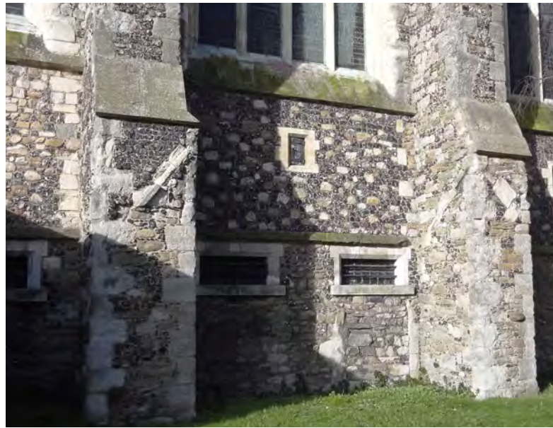
(a) Detail of 1867 cell windows, ventilation hatch and mediaeval porch(?) marks on buttress. (Internal ref: DSC05638)
