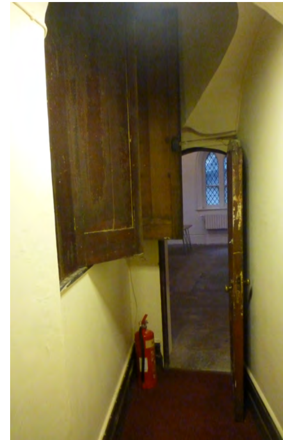
(f) Base of spiral stair remains behind cupboard doors in corridor. (Internal ref: P1110071)
