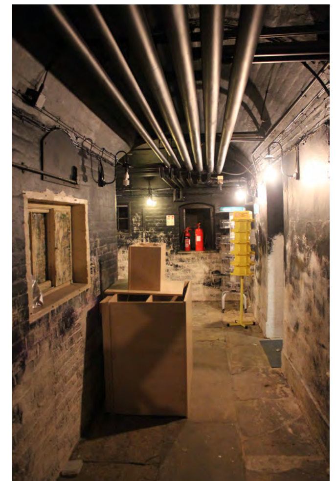
(e) West side of Stone Hall undercroft. (Internal ref: DSC05495)
