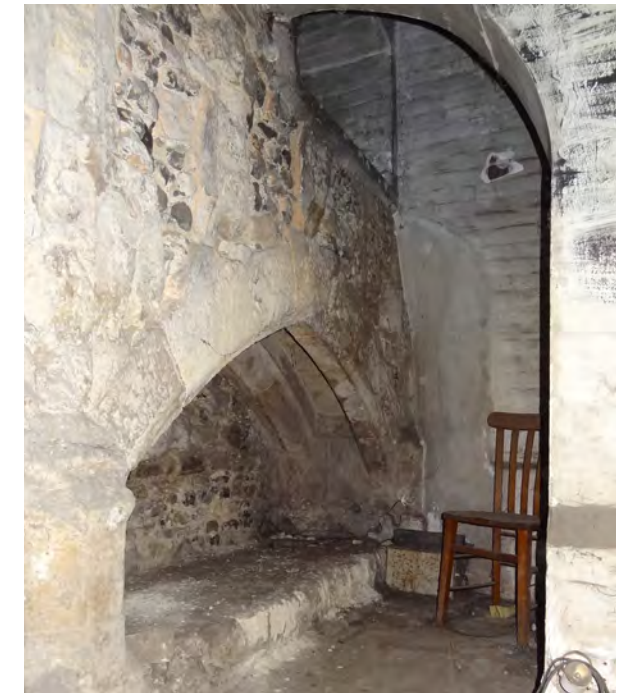
(e) Earlier floor level shown within cell with surviving tombs and steps up to the 1835 prison floor. (Internal ref: DSC05505 & DSC05518)
