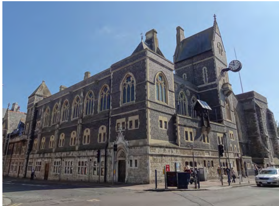
(a) Dover Town Hall at corner of Ladywell and High Street. Connaught Hall and Clock Tower in the foreground with Mediaeval Tower in the distance. (Internal ref: DSC03174)
