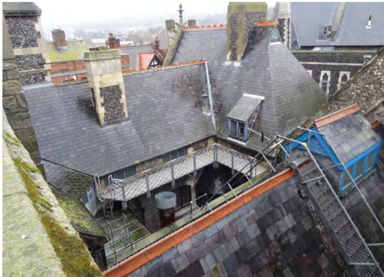
(a) Roofs to Mayor's Parlour Suite (Internal ref: DSC05010)
