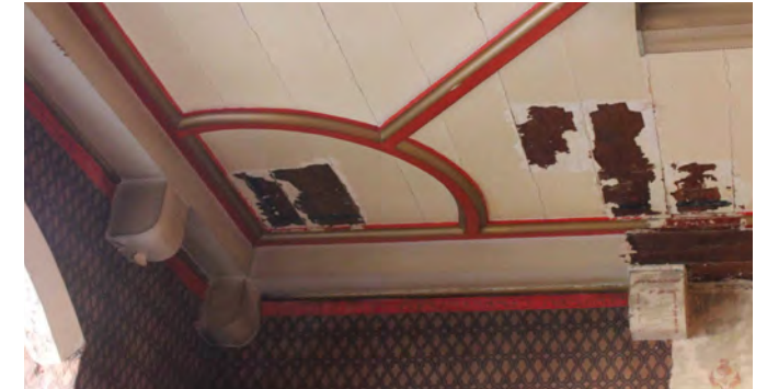
(e) Ceiling to Mayor's Parlour Office (FF) (Internal ref: IMG_5972)
