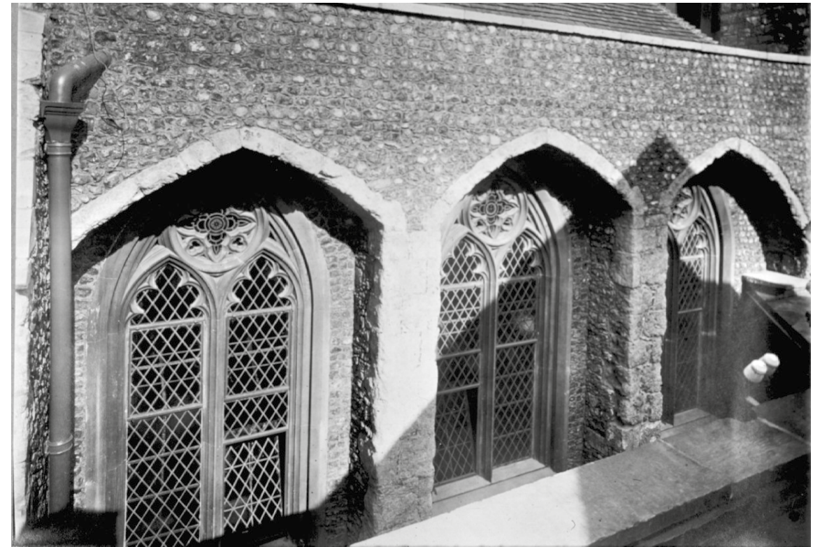
(c) South wall of Sessions House showing mediaeval relieving arches between buttress piers. (DMA ref: D02025)
