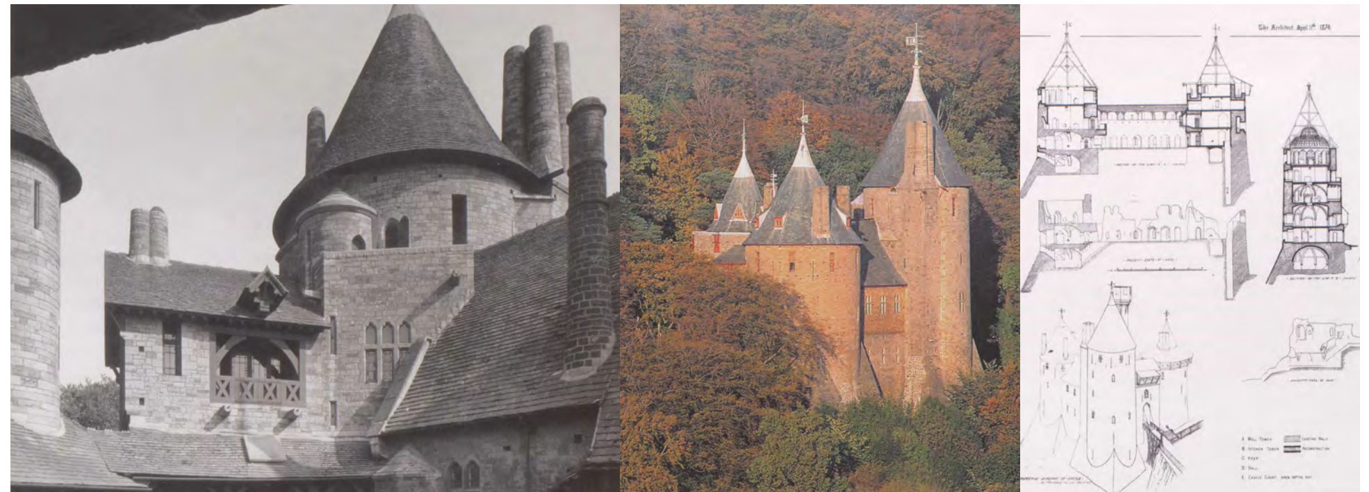
(b) Photographs and drawings of conical roofs and chimney shapes at Castel Coch, by Burges. Similar conical roofs can be found at Dover Town Hall. See Plate 12(c) and Plate 26(j) (Internal ref: J Mordaunt Crook_266, J Mordaunt Crook_268, J Mordaunt Crook_265)
