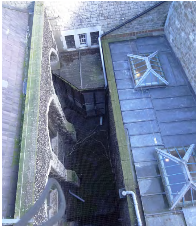
(b) Courtyard between Sessions House and Council Chamber (Internal ref: DSC05586)
