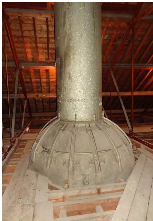
(d) Sun Burner funnel. Galvanised riveted plates but still with Gothic decoration. (Internal ref: DSC04988)
