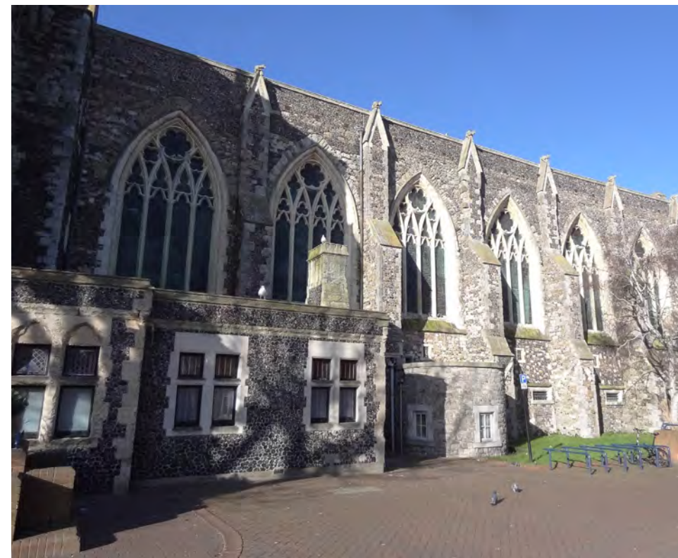
(e) South side of Stone Hall (Internal ref: DSC05653)
