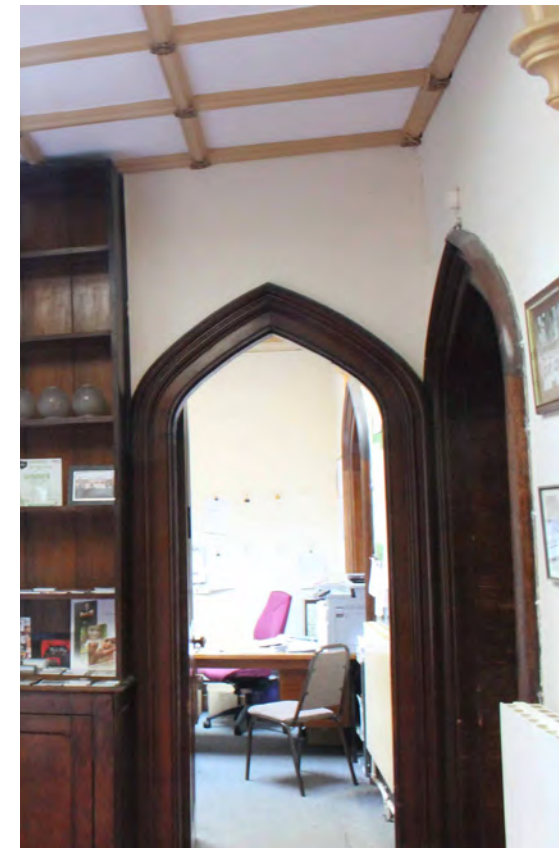
(g) Pointed arched doorways with deep reveals to ante-rooms. (Internal ref: IMG_7076)
