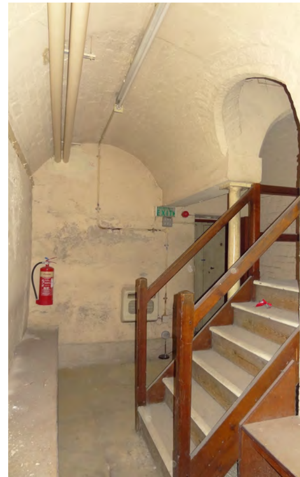
(g) Timber stair leading to Sessions House (Internal ref: DSC05542)
