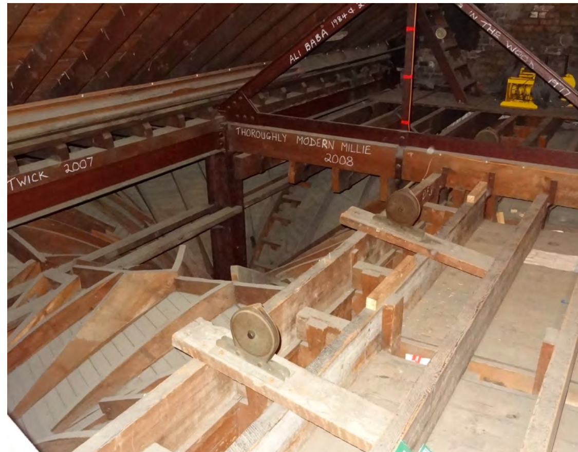
(e) Detail of timber boarded vaults over gallery. Note pantomime production titles. (Internal ref: DSC04992)
