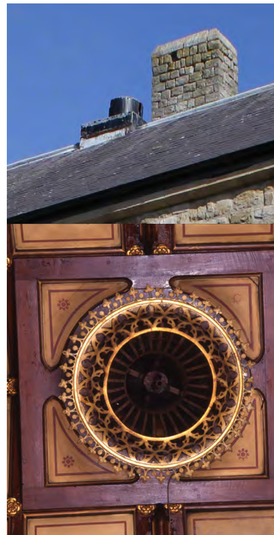
(d) Sun Burner to Council Chamber and simple rooftop ventilator. (Internal ref: IMG_4677 & DMA ref: d23403)
