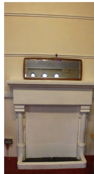
(g) Picture rail 'banding' & domestic fireplace (Internal ref: IMG_7945)
