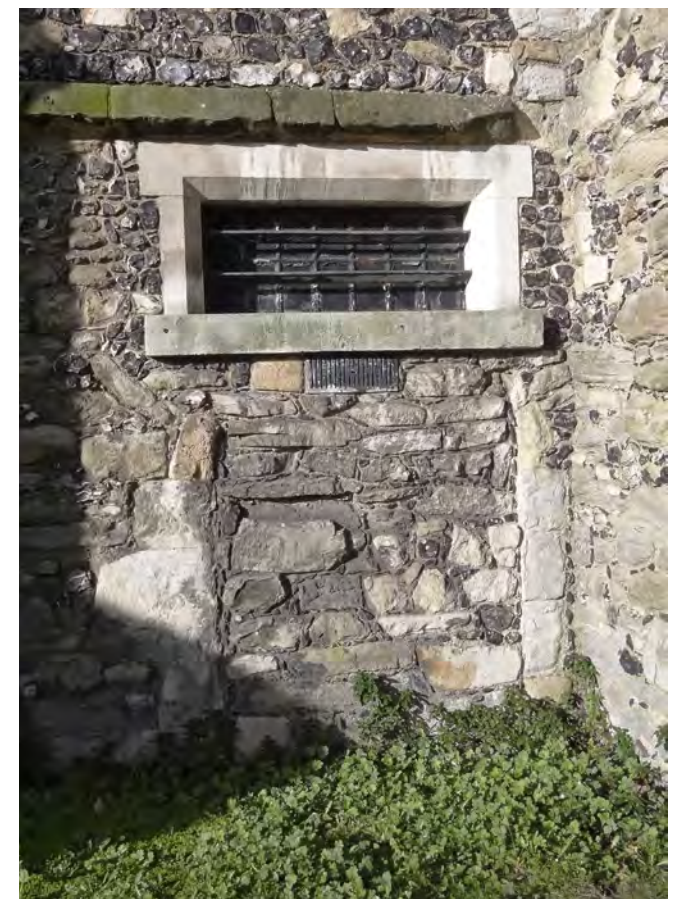
(f) Now blocked doorway to Stone Hall (Internal ref: DSC05641) [Refer to App.01_Fig.2.5]
