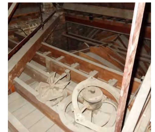
(g) Disused Sun Burner fans and funnel above. (Internal ref: IMG_4638 & DSC04985)
