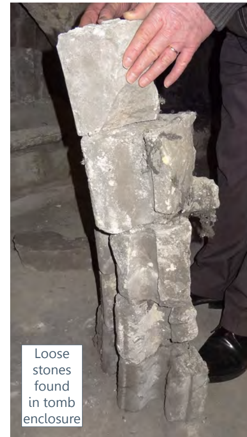
(d) Stacked stones form deeply moulded arch surround. (provenance unknown) (internal ref: DSC05520)
