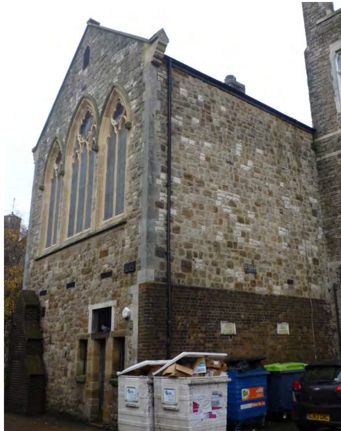
(a) East wall of Council chamber sits on prison yard wall (Internal ref: P1110066)
