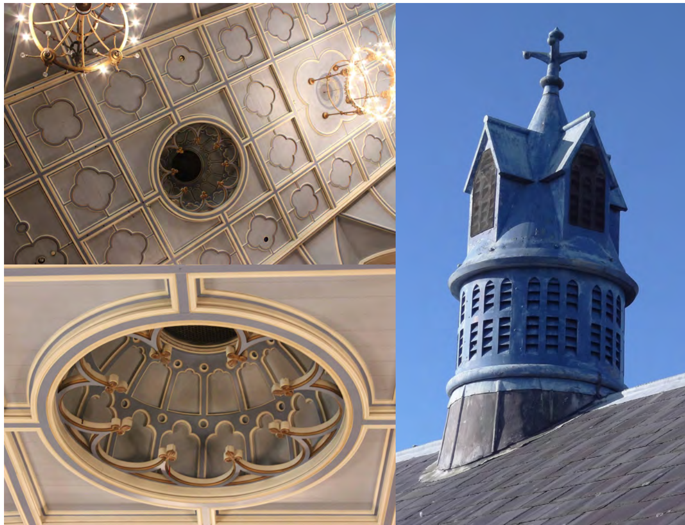
(a) Details of the surviving moulded, domed funnels to the Connaught Hall sunburners with detail of roof cowl. (Internal ref: IMG_7108, IMG_7563 & DSC05625). Refer to Plate 15(d) and (g) also.
