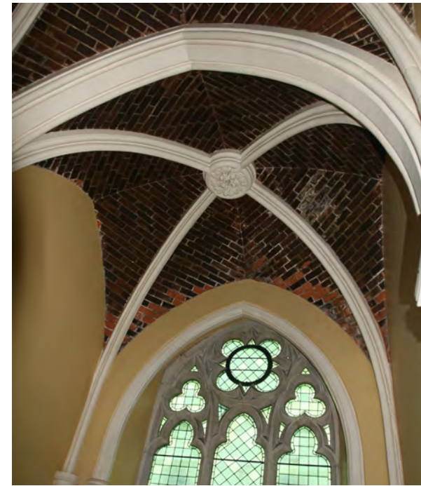
(d) Brick vaults and windows to stairwells (Internal ref: IMG_4707)
