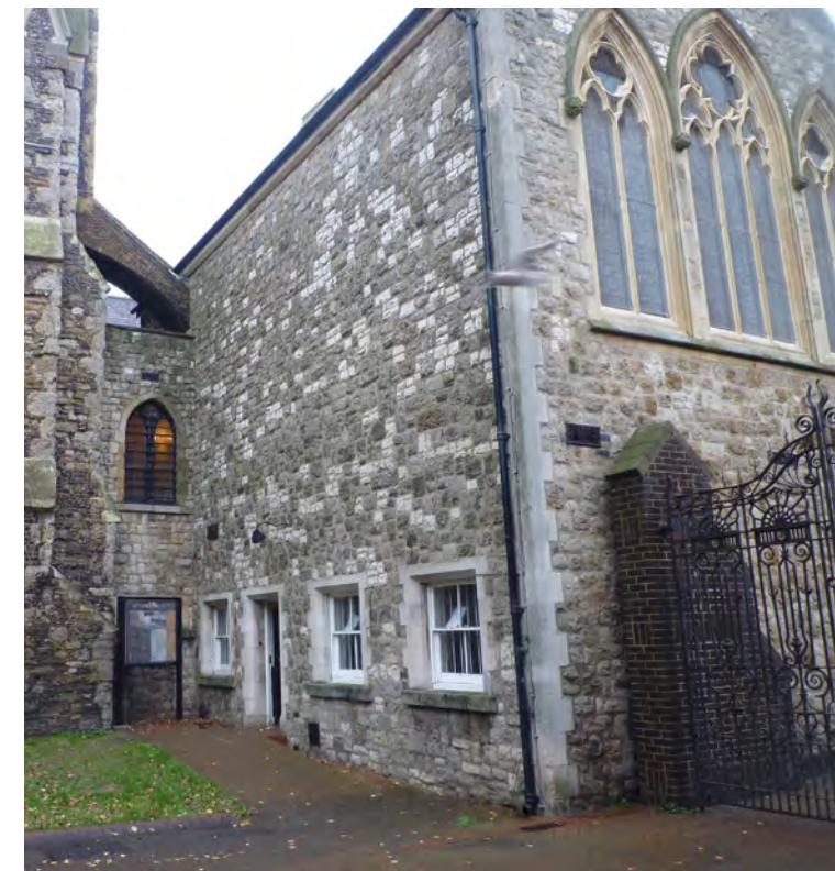
(f) Council Chamber south and west sides. (Internal ref: P1110063)
