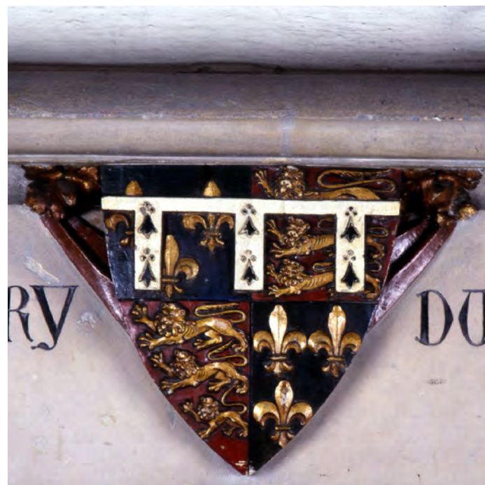
(f) Shields to Stone Hall below the dado string course. The painting is discussed in Burges correspondence. (DMA ref: d11725)
