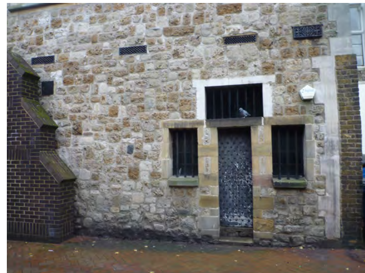
(c) Original entrance to day cells below Council Chamber (Internal ref: P1110064)
