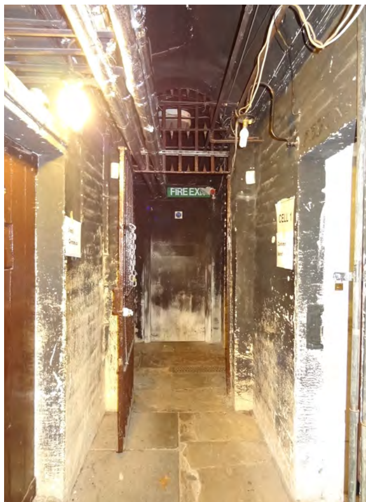
(c) Gaol cells under Stone Hall (Internal ref: DSC05495)
