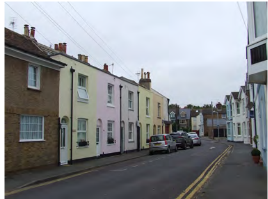
A terrace within the conservation area
