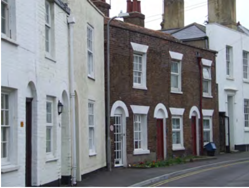
A row of terraced buildings within Wellington Road
