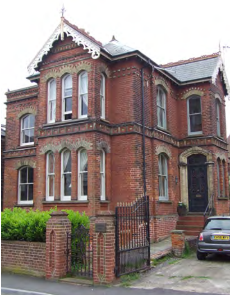
Wellington House is a prominent building within the street
