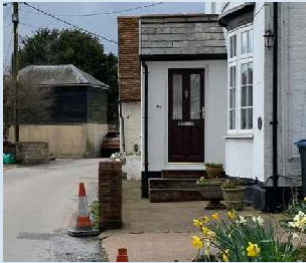
Slate roof pitched roof porch
