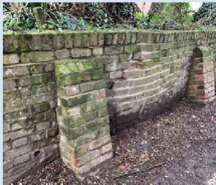
Brick wall with buttress
