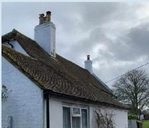
Clay tile cat slide roof
