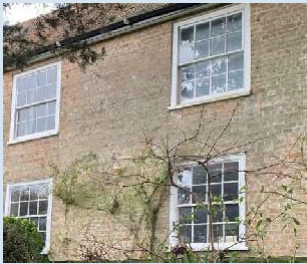
Sash windows with light frames
