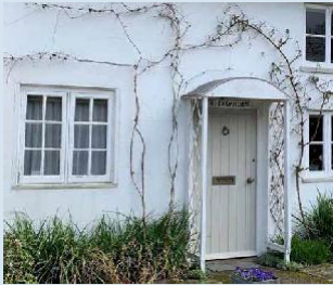
Wooden casement windows and wooden panel door
