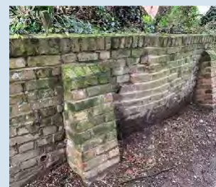
Brick wall with buttress
