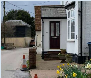
Slate roof pitched roof porch
