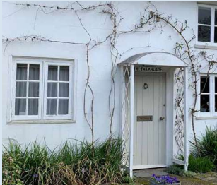
Wooden casement windows and wooden panel door
