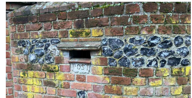
Figure 92: Flint and brick wall in East Langdon.
