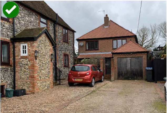
Figure 87: Good example of a side extension which respects the roof pitch, materials and scale of the original building.
