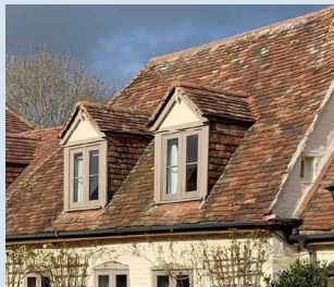
Kent peg tiles in light/ red brown and gabled dormers
