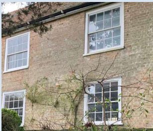
Sash windows with light frames
