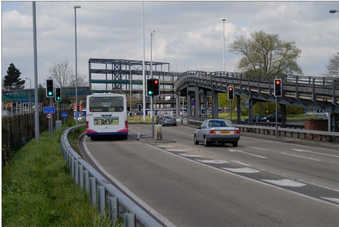
Figure 6.13 – Bus Priority Signals to stop general traffic and allow buses through
