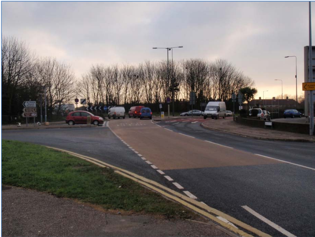
Figure 6.9 – Sandwich Road on the approach to the roundabout with the A2
