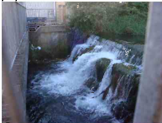
Weir and culverts constrict the River Dour
