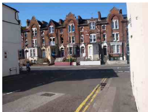
Looking towards basement properties on Folkestone Road from Malvern Road
