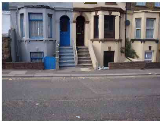
Low thresholds to basement properties at the bottom of Coombe Valley Road
