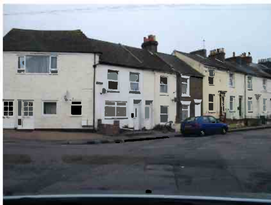
Basement properties in West Street ponding area
