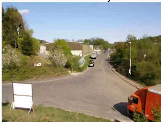
Depression in Poulton Close before road continues to slope steadily downwards
