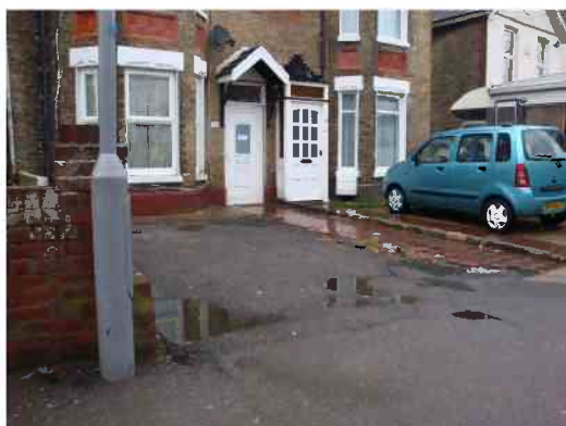
Low property thresholds at junction of Folkestone Road and Elms Vale Road
