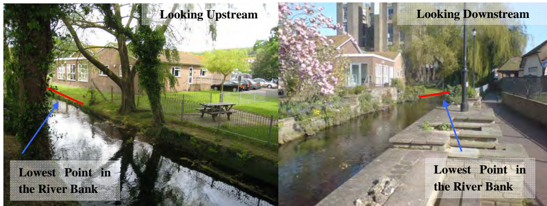
Figure 4.5 Location of lowest bank elevation (red line) within the Mid Town Site
