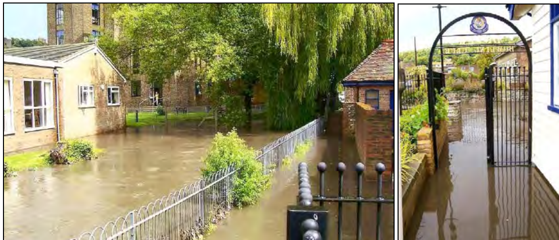
Figure 4.20 Photos of River Dour within the Mid Town Site Taken After the June 2007 event. (Source: JBA consulting)
