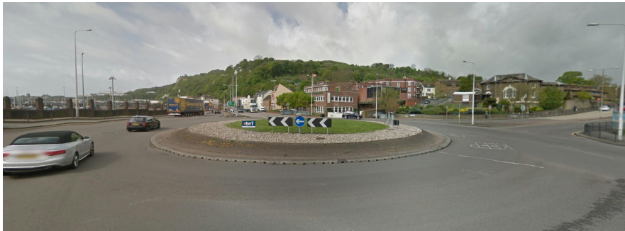
View toward the Drop Redoubt from the A20 near the harbour (copyright Google 2014)
