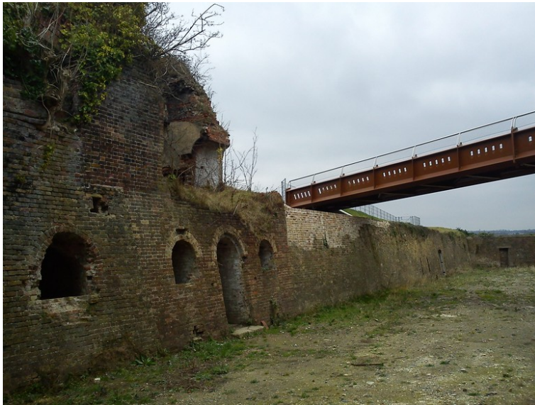
New bridge, Fort Amhurst Chatham (photograph taken by Colin Godfrey)
