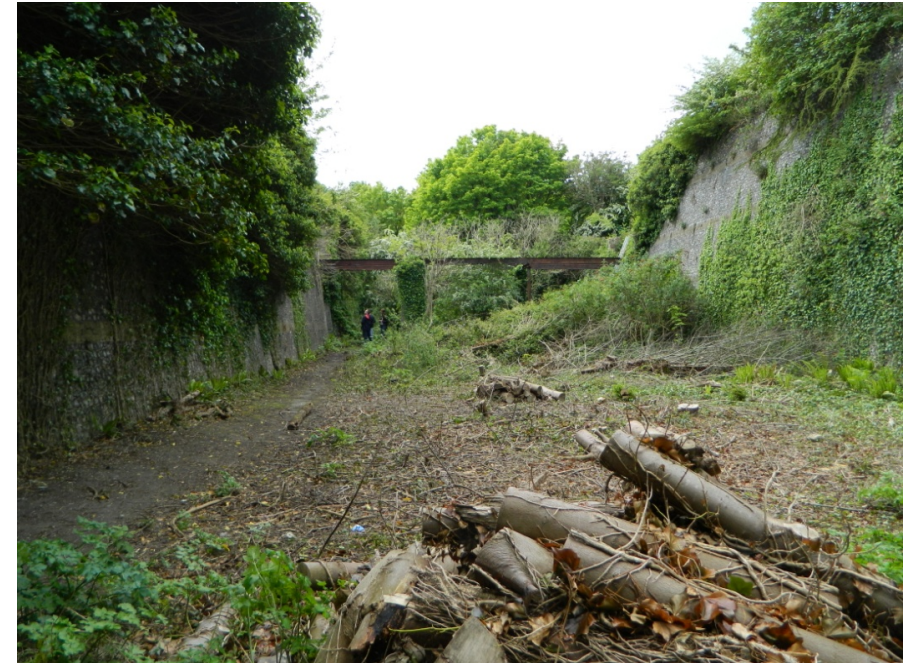
Subterranean defensive works that lie beneath the colonising mantle of invading vegetation
