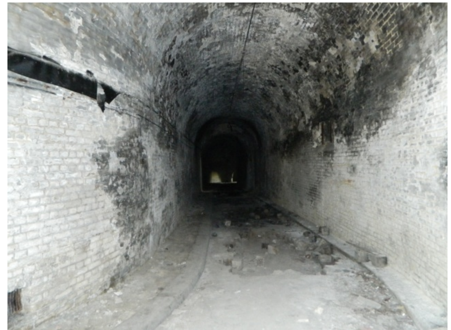
The North Entrance Tunnel
