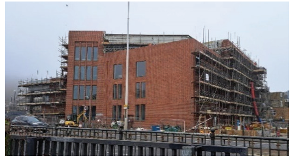
Figure 3 - The Bench viewed from Townwall Street looking North-West
