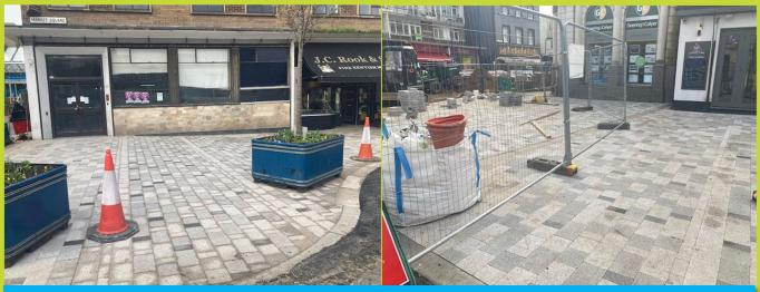
Paving being laid in the Market Square will be cleaned and sealed to prevent staining in the coming weeks.
