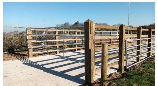
Image above shows Installation of fencing for Cattle crossing.
