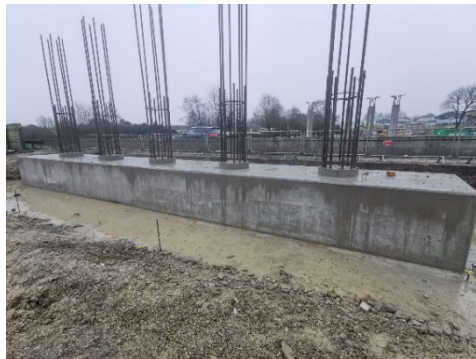
Image above of the Construction Pile cap in Section 1B North
