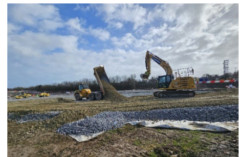
Image above of Embankment fill in Section 1B North.
