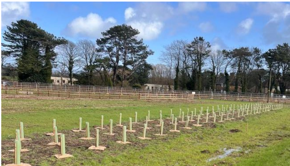
Image shows a section of the planting being carried out in Section 2
