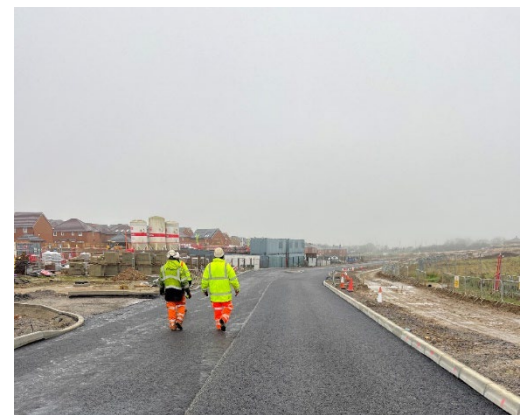
Image shows the first layers of tarmac in Section 1a/1b North.
