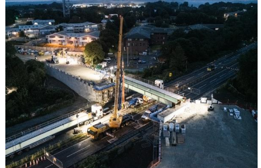
Above: Image of Bridge Beam lift
