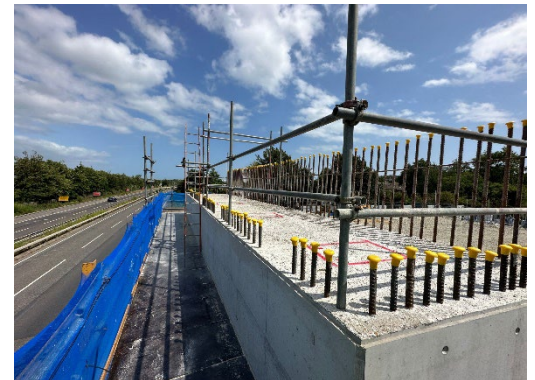
Image: Crosshead in Section 1B south
