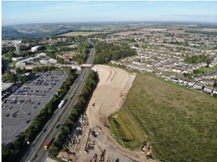
Image above shows view towards bridge and embankment.
