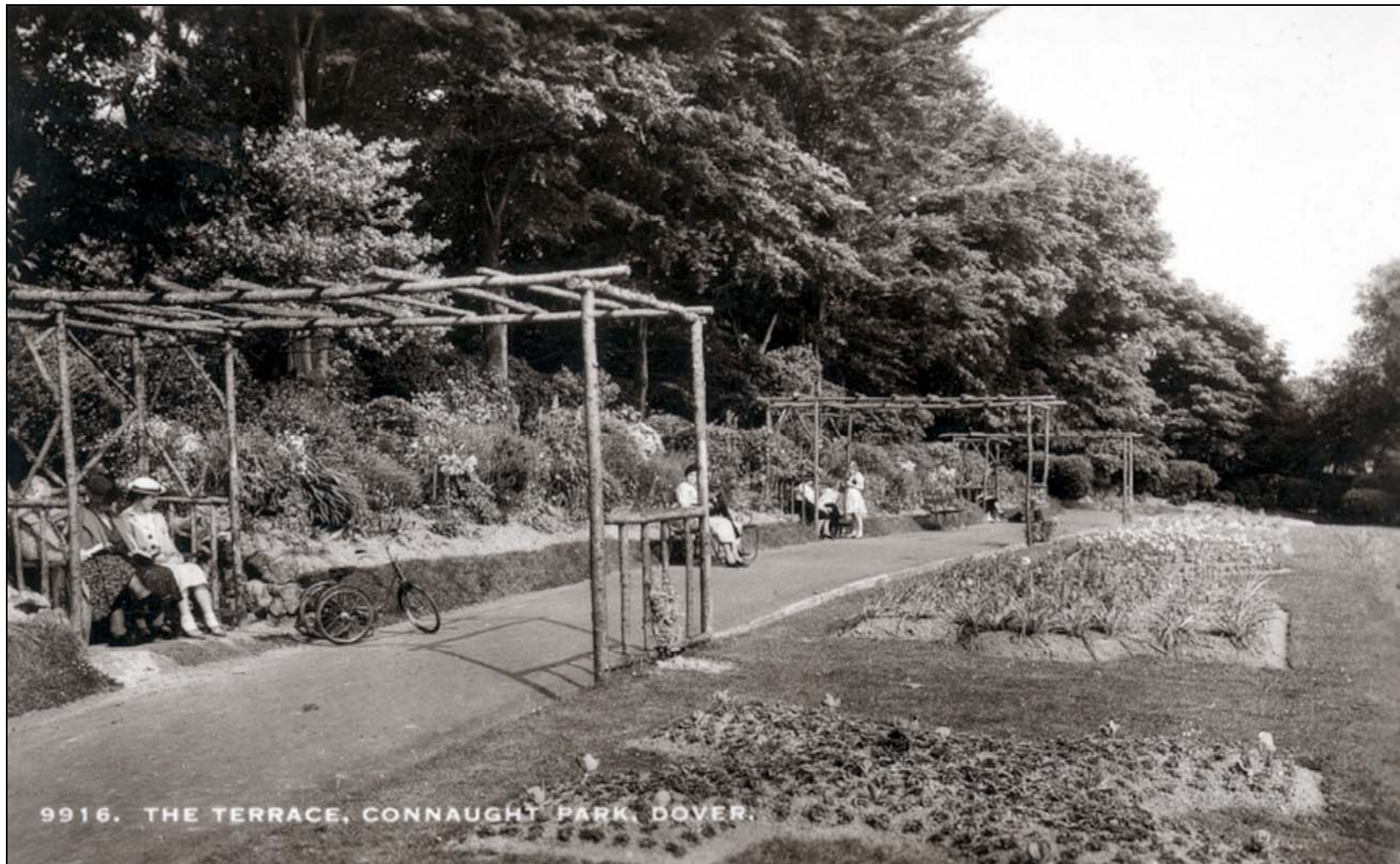
Fig. 10 Photograph of Connaught Park Terrace 1933 (courtesy of Dover Museum)
