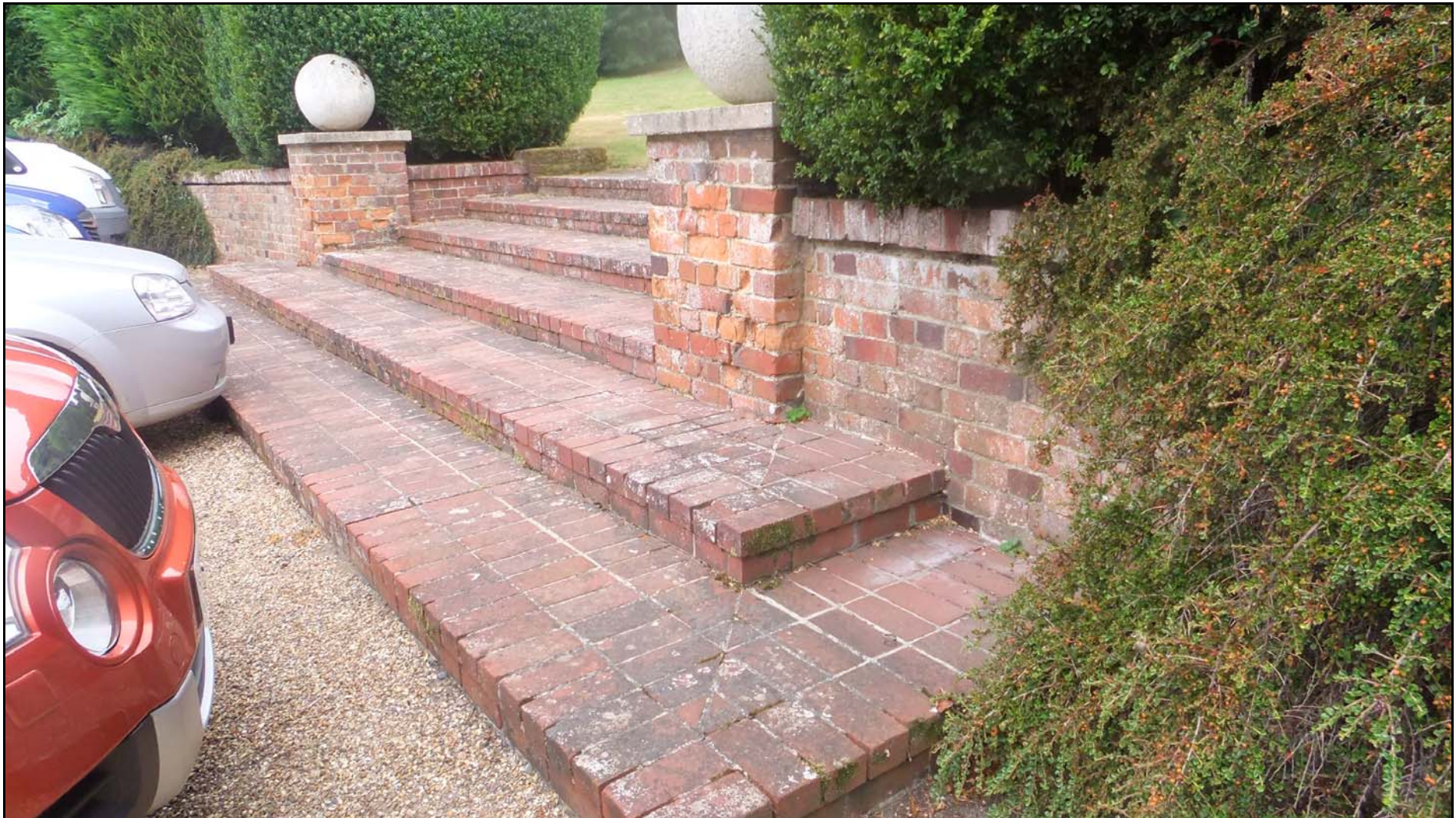
Fig. 16 Steps opposite West Façade (2016)
