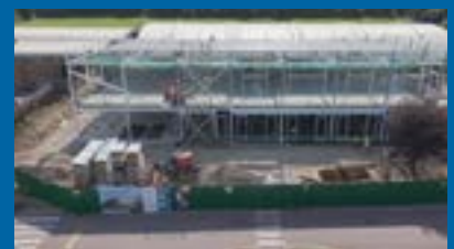
Figure 1: The new Deal Leisure Centre swimming pool under construction.
